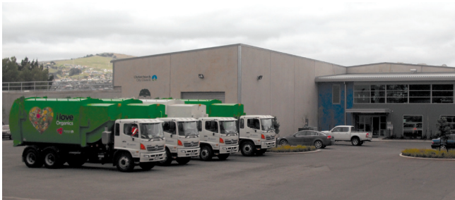
Living Earth's Organics Plant
