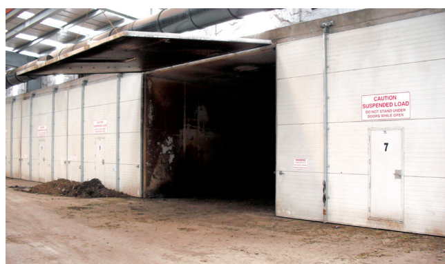
Enclosed tunnel for 21 days
