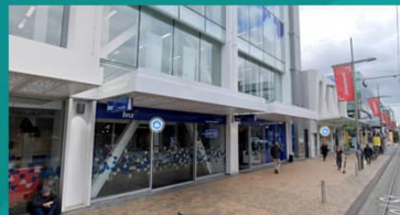
structures on streets
