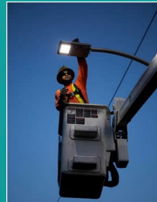
street light maintenance
