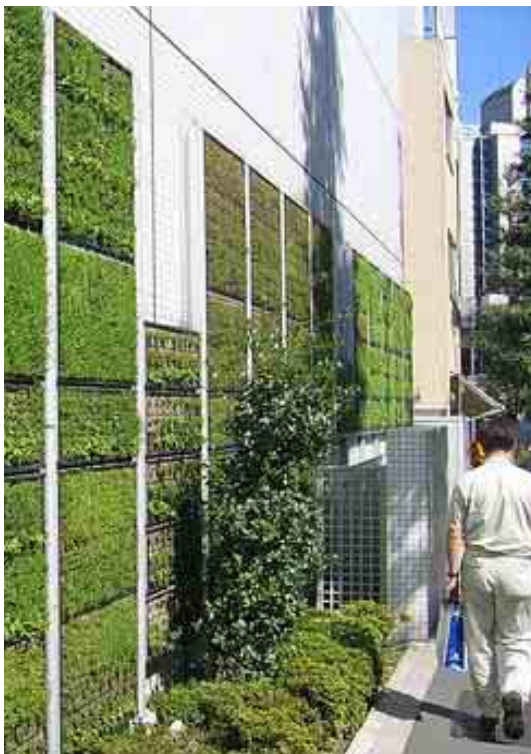
'Green walls' soften lane edge (London)
