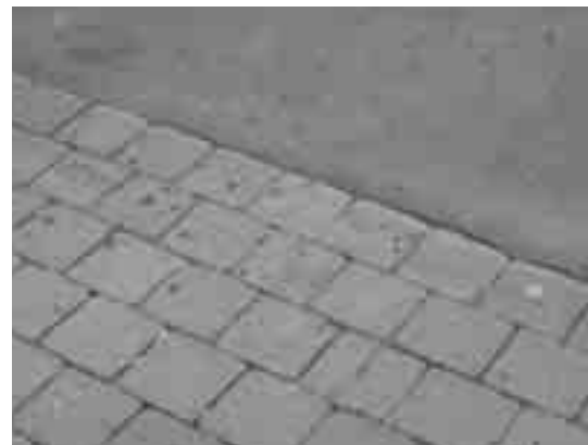
Sett pavers with asphalt surfacing
