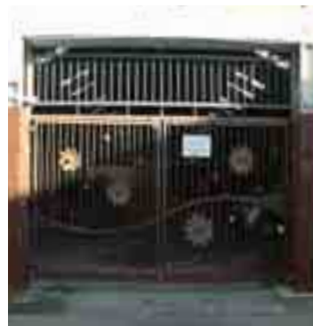
Gates should be considered as a design item (Ash Street)
