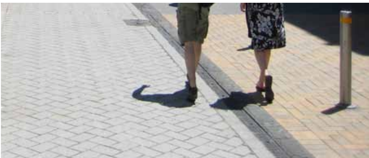
Paving, City Mall
