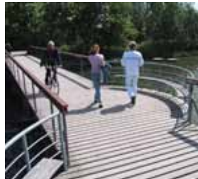
Pedestrian and bicycle bridge with sitting opportunities. Copenhagen, Denmark
