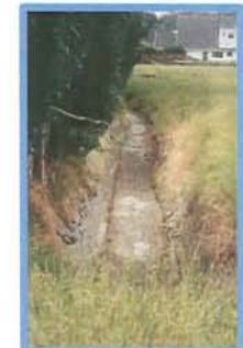
Cracraft Historic Drain
