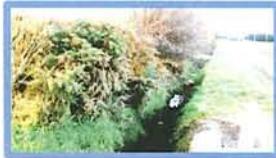
Drain along Sparks road
