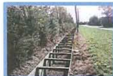
Channelised Drain alongside Sparks road
