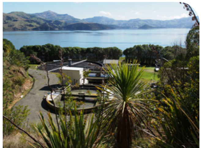
Akaroa wastewater treatment plant
