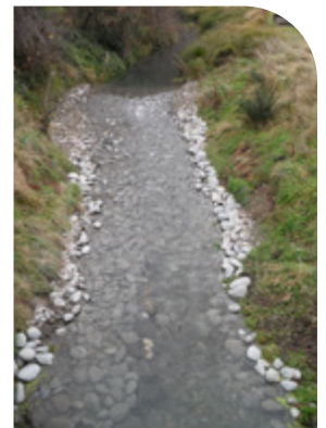
Knights Stream restoration added riffles and fish passage
