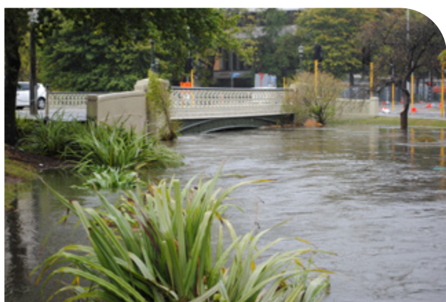
Ōtākaro Avon River flooding, March 2014
