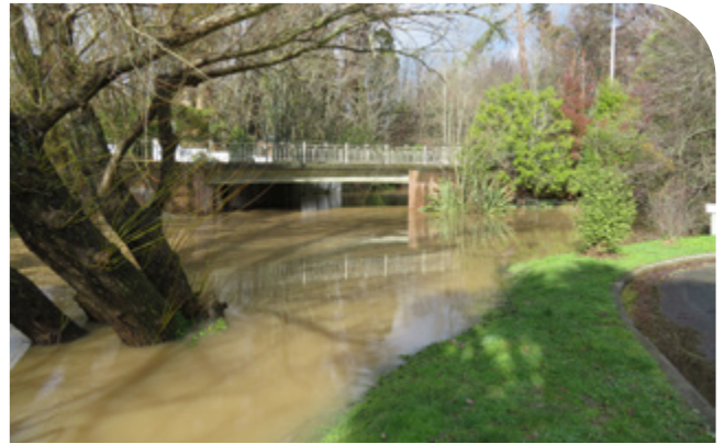
Flooding on Ōpāwaho Heathcote River in Somerfield 2017
