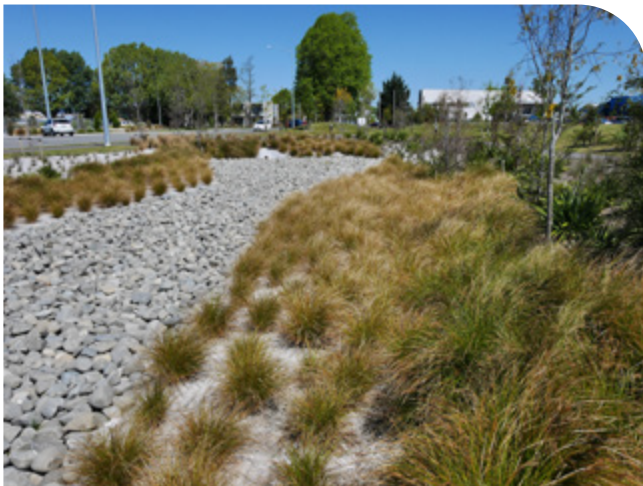
Stormwater control, Tait Industrial Park
