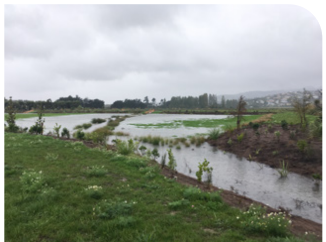
Eastman Wetland, constructed stormwater basin, detaining stormwater
