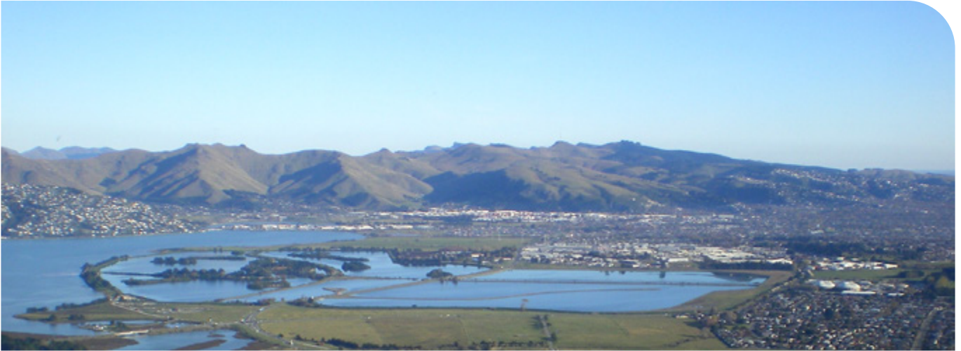
Aerial view of Bromley oxidation ponds
