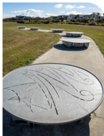
Retention basin drainage covers at Wigram Skies
