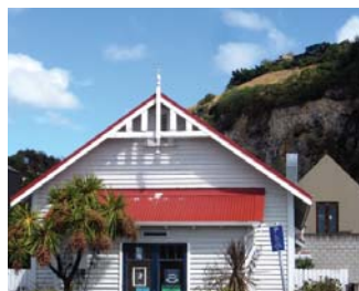
Detailing within the roofscape
