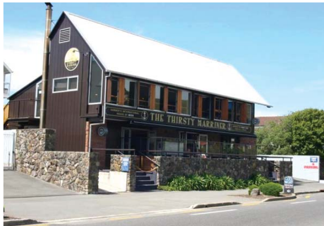
The former 'Thirsty Marriner' Public House; Marriner Street. An example of dealing with level change within the plot through the creation of usable spill-out space along the street.
