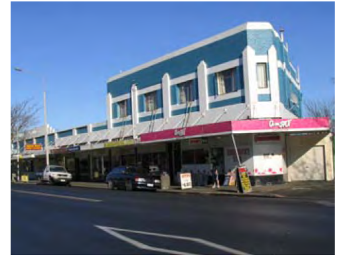
Figure 1. Part of the Selwyn Street shops in 2005
