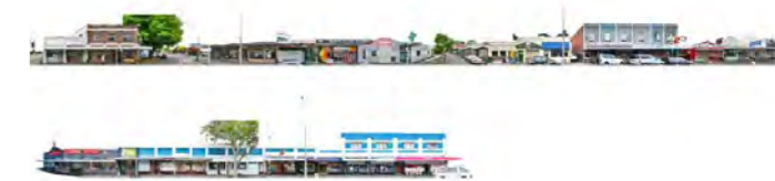
Figure 11. Pre-earthquake street frontage (from 2009)
