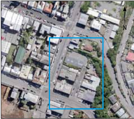
▲ Council owned property in Donald Street.
