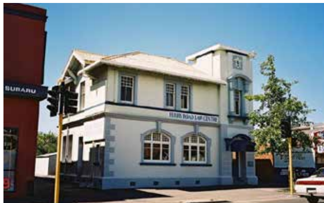
Figure 99 - Ferry Road Law Centre (697 Ferry Road).
