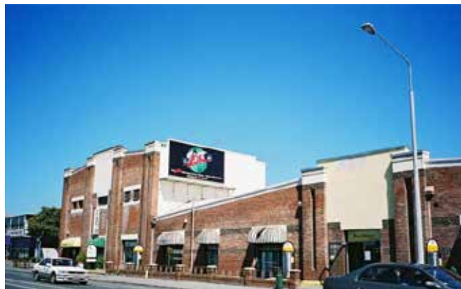
Figure 98 - A&T Burt Building – former Nugget Boot Polish factory (580 Ferry Road).
