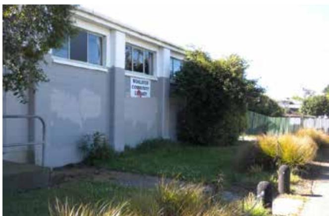
Figure 89 - Woolston Community Library relocated after demolition of their original facilities.
