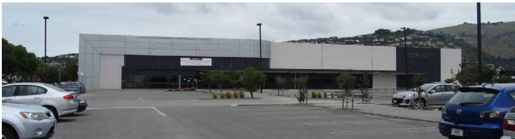
Figure 82 - Ferrymead Countdown before demolition (see Issue E5).
