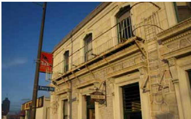
Figure 96 - Lancaster Hotel (184 Ferry Road).
