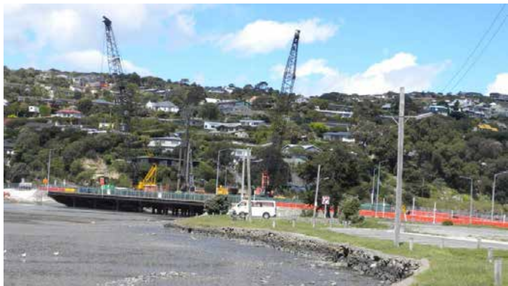
Figure 21 - Ferrymead Bridge repairs, October 2013.
