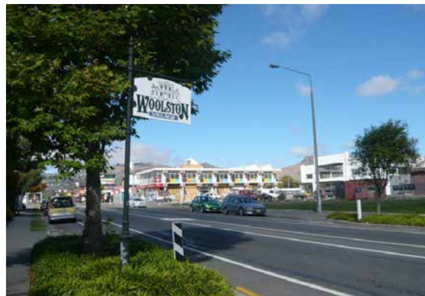
Figure 59 - Current gateway at western entrance to Woolston.
