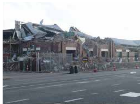
Figure 19 - Demolition of the former Nugget Boot Polish factory at 580 Ferry Road.
