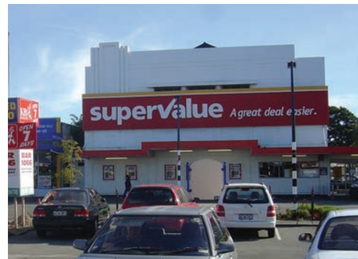
Figure 2g – SuperValue supermarket in the former Century Cinema building (photo taken: 2009).
