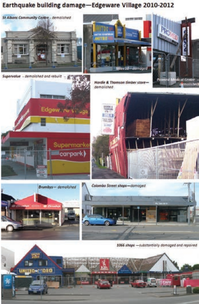
Figure 2r – Images of earthquake damage to buildings.
