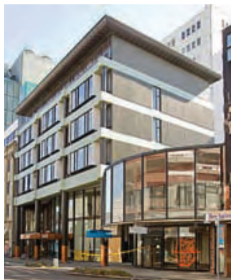
2: Building before Demolition
