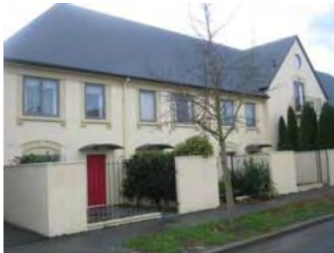
Photo 1: Chester Street East
