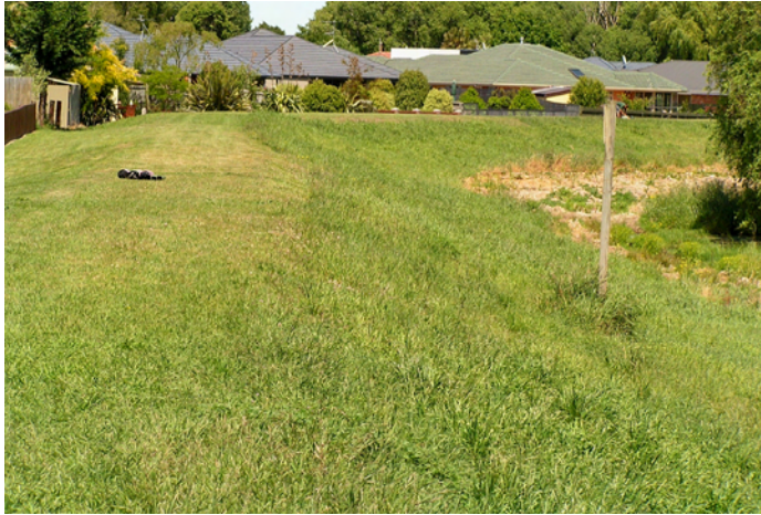
Figure 1 Stopbanks such as this one modify the natural character of the landscape. They do however denote the landscape processes that prevail in the area – in this case the risk of flooding.
