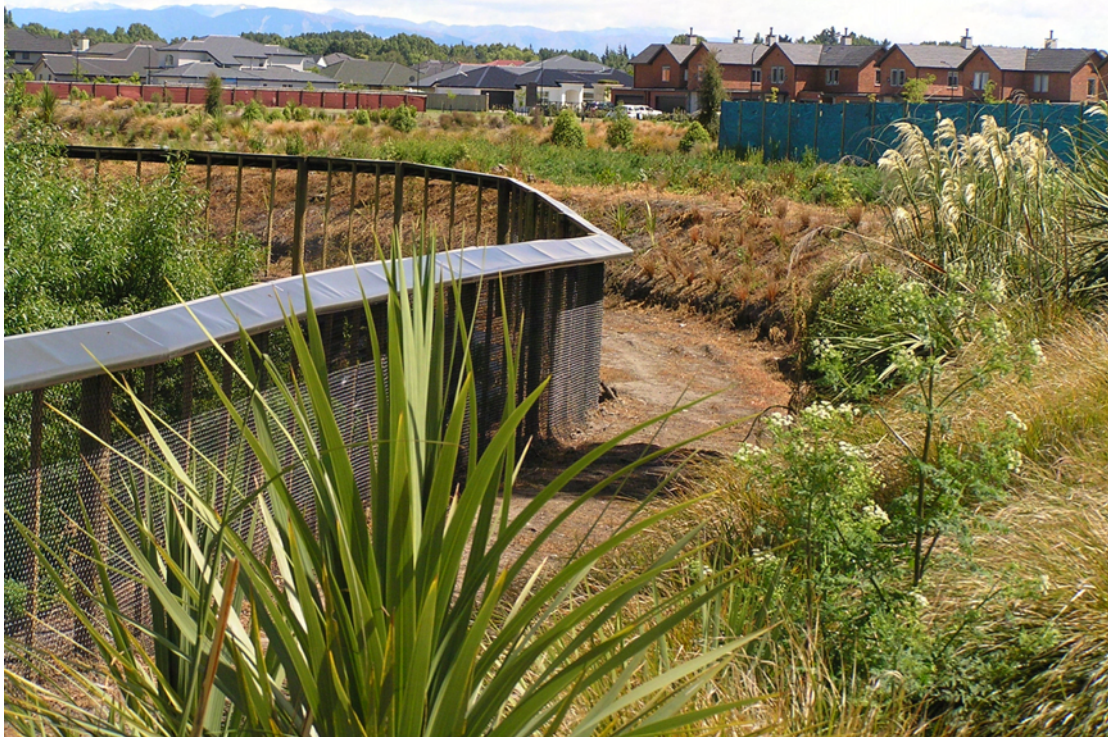
Figure 38 A predator proof fence at Northwood is a good example where urban development happily coexists with the realisation of conservation objectives.
