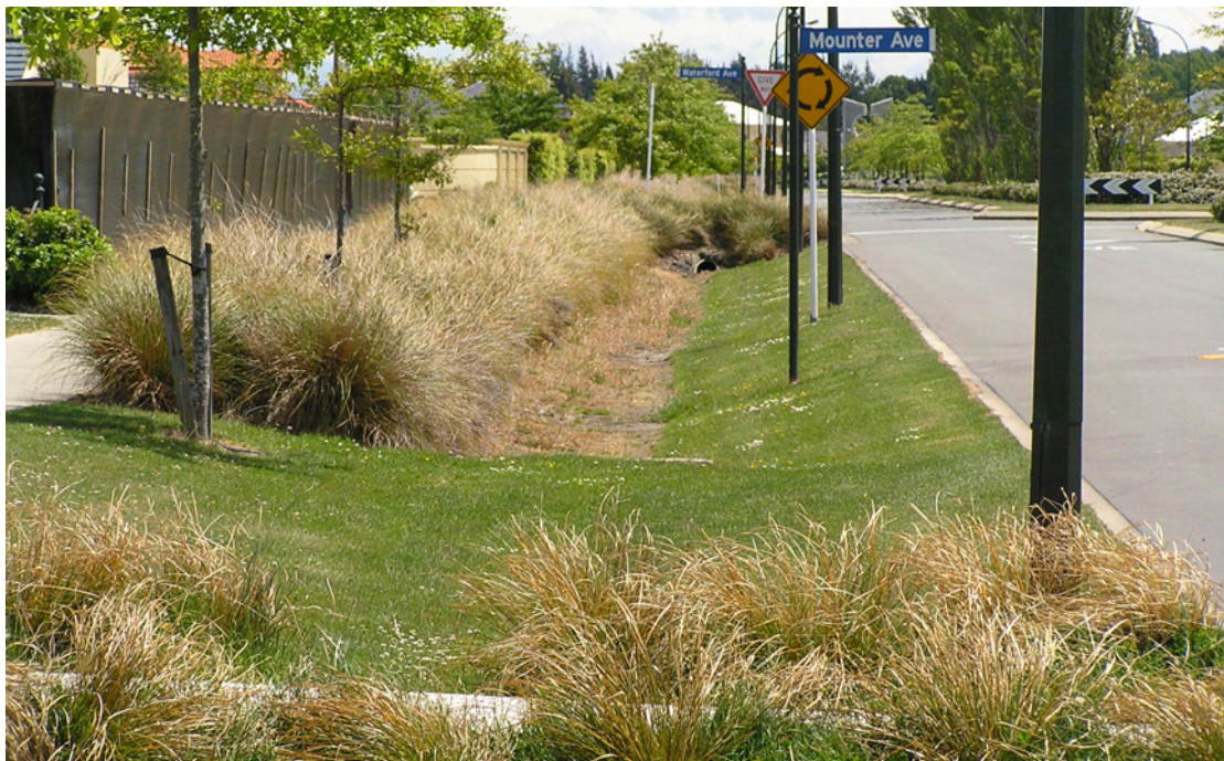
Figure 37 A good example at Northwood of integrated stormwater management, pedestrian footpaths and roadway with a mix of exotic and native planting.
