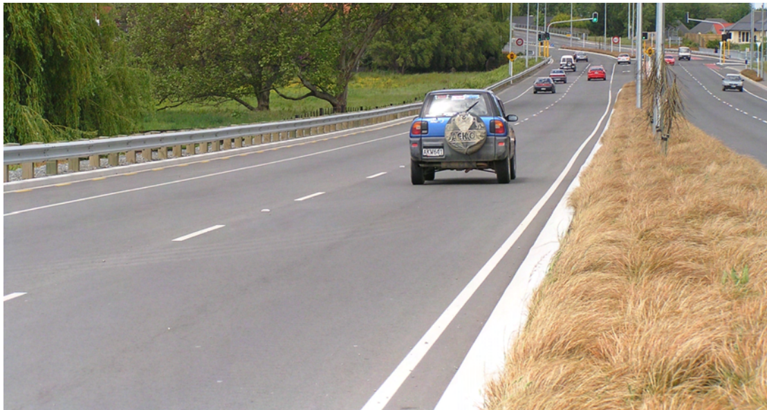
Figure 11 Native planting in the road median between Styx overbridge and Johns Road.
