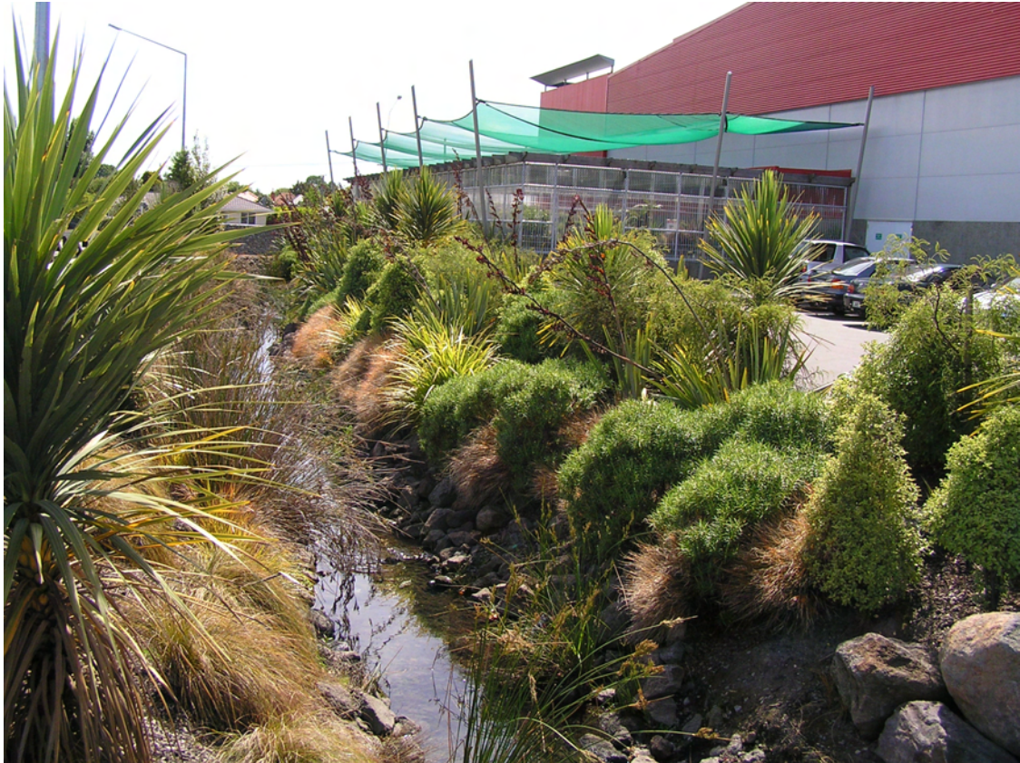
Figure 53 A good example of integrated stormwater drainage and ecological restoration with large scale commercial development – in this case at Northlands Mall.
