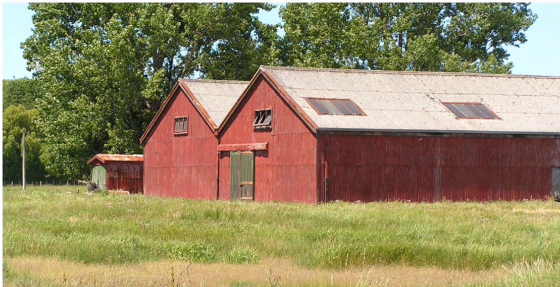
Figure 42 These old buildings on Belfast Road may have potential for reuse as community facilities such as an arts cooperative or for indoor sports. The surrounding land could be used for a park in the vicinity of freezing works.
