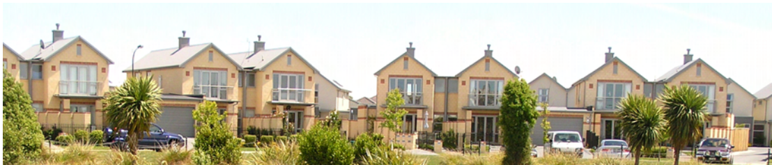
Figure 28 Enclaves of high density housing (L3) is a feature of Northwood subdivision which adds to living zone diversity in the Belfast area.
