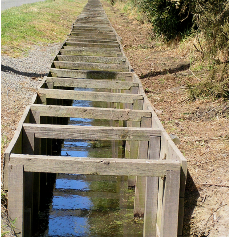
Figures 43 & 44 Boxed drains are still relatively common in the Belfast area. If sufficient space is available there is potential to naturalise them so as to create a more ecologically friendly environment such as that shown below.
