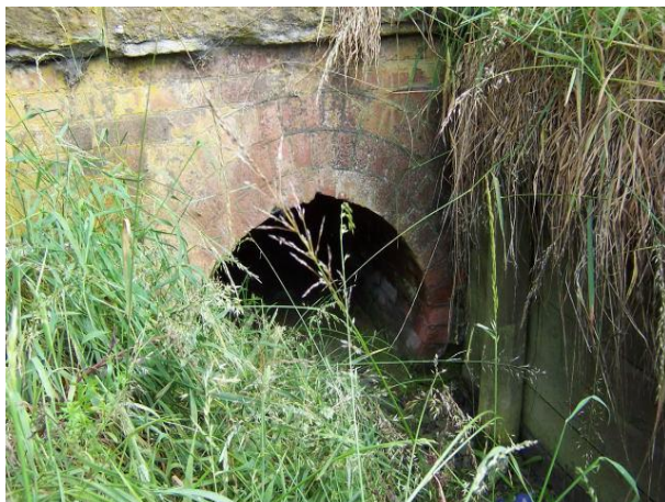
Railway culvert adjacent to Marshlands Road
