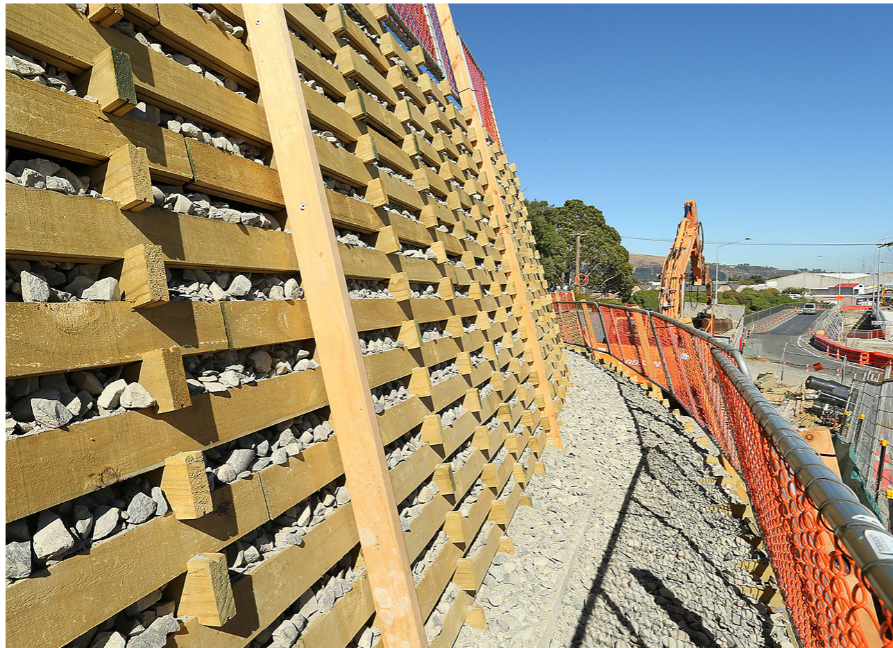
Construction work near Ferrymead Bridge.
