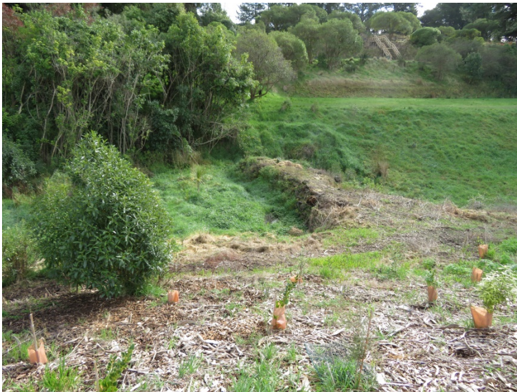
Source: T Ussher April 2017. The upper weir with the breach on the far, north side visible.
