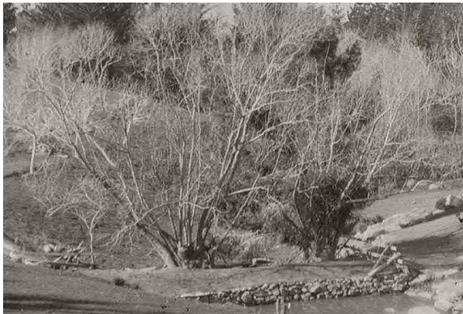
The upper weir c1890
