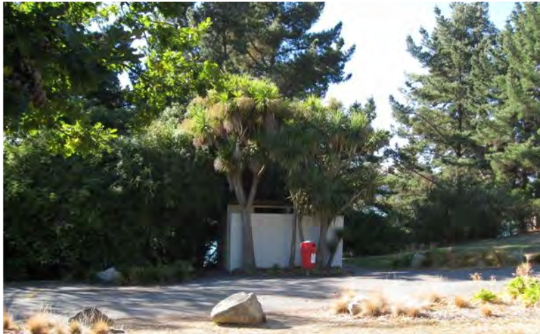
Stoddart Point picnic area toilet block, hidden by surrounding vegetation. Photo taken in April 2010.
