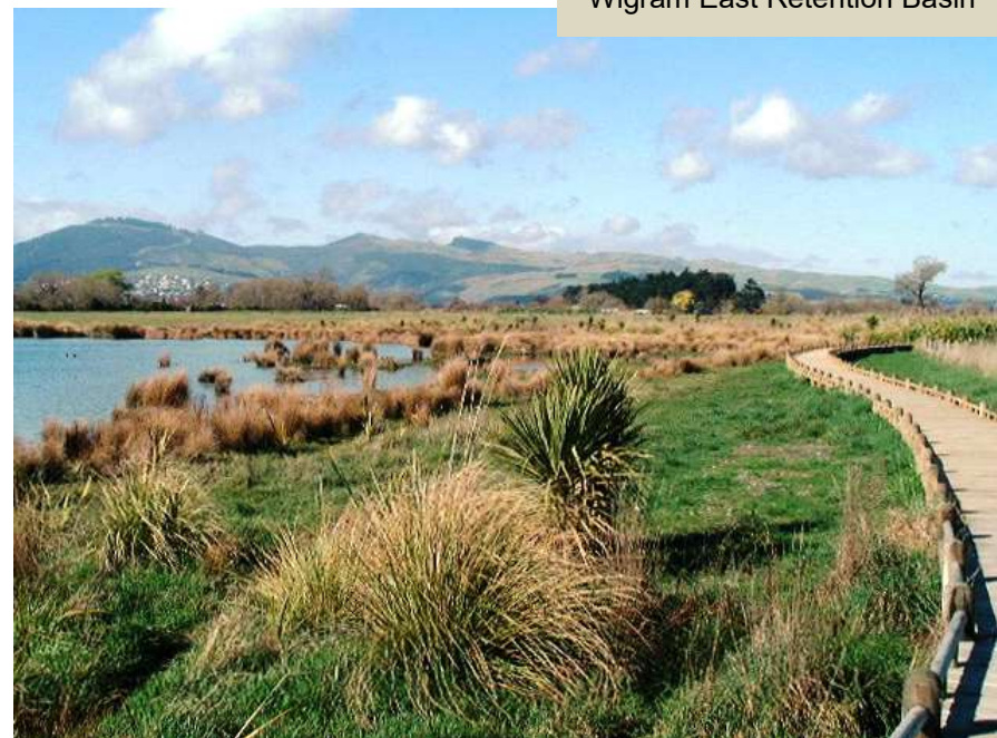
Wigram East Retention Basin
