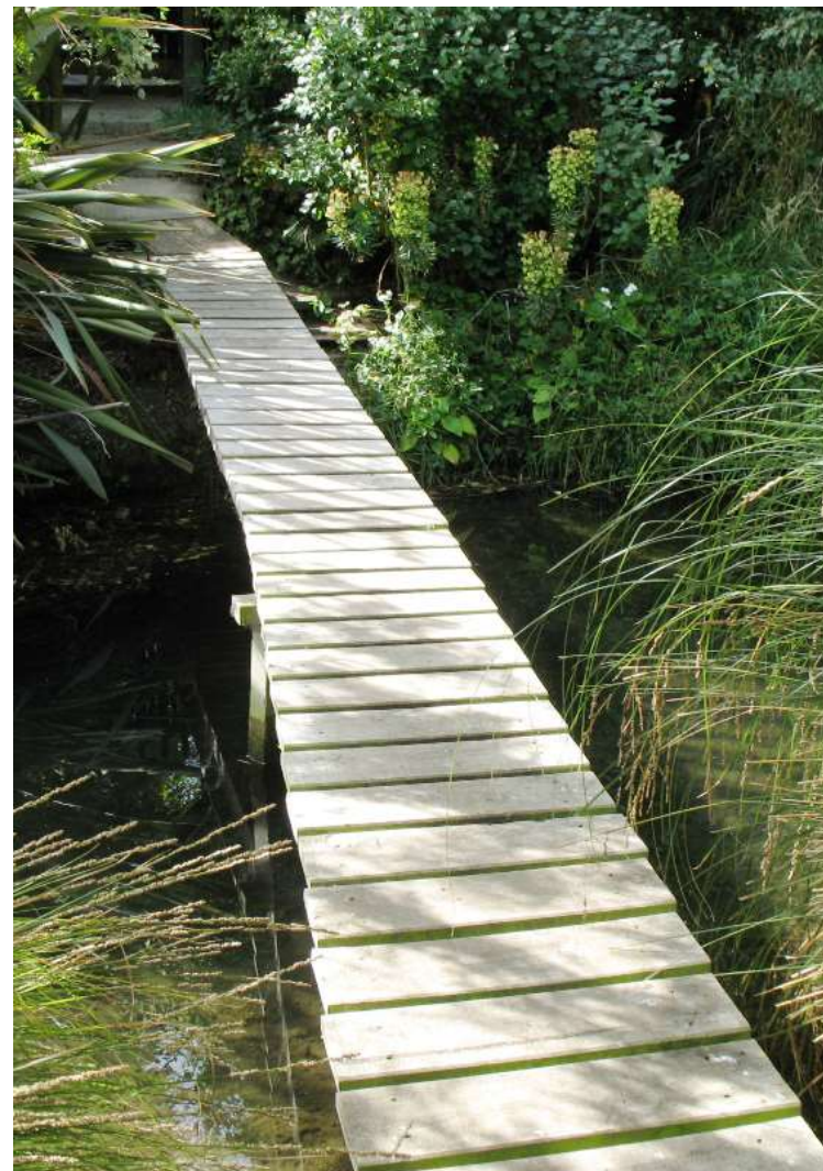
Boardwalk bridge over the Heathcote River/Ōpawaho – Ngā Puna Wai
