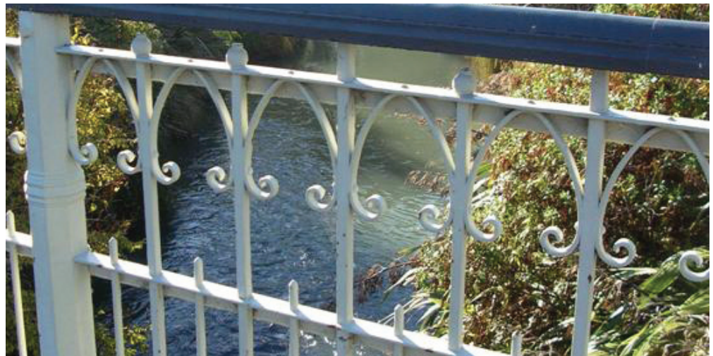
Historic bridge detail on Colombo Street bridge.
