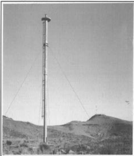
Wind Generator (without propeller), Bowenvale Park
