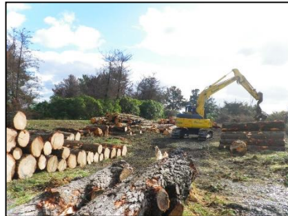
Tree removal in Bridge Reserve 2012
