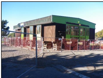
Transitional community building being put into place
