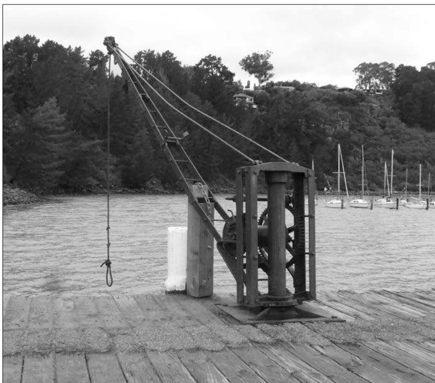
Diamond Harbour jerry crane, 2016. P1150359, L. Beaumont
