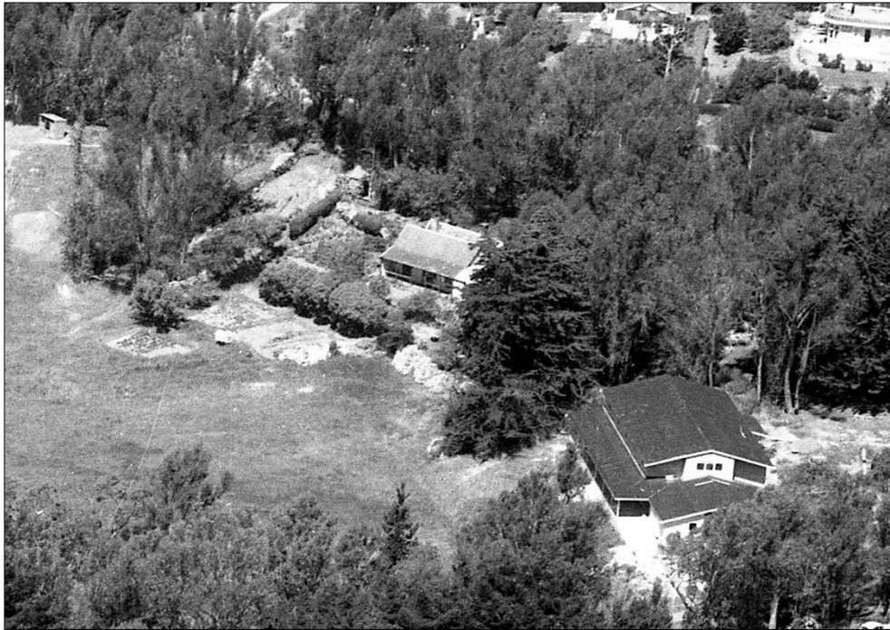
Figure 22: Aerial view of Stoddart Cottage and the Memorial Community Hall under construction, 1954 Note the density of planting in the cottage garden and boundary hedge on east of the property Source: 1473-1502 V C Browne & Son
