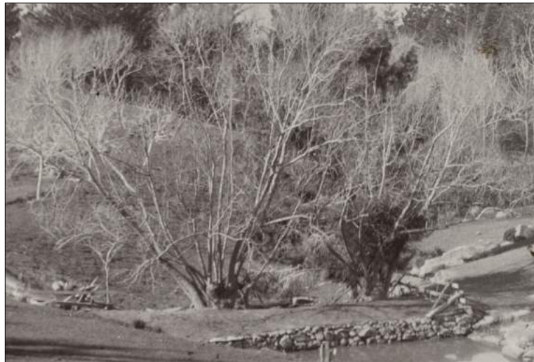
Figure 6: Stoddard weirs and weir detail, c. 1890s Source: 2015.114.75, Stoddart Album 1, Page 16, CMDRC
