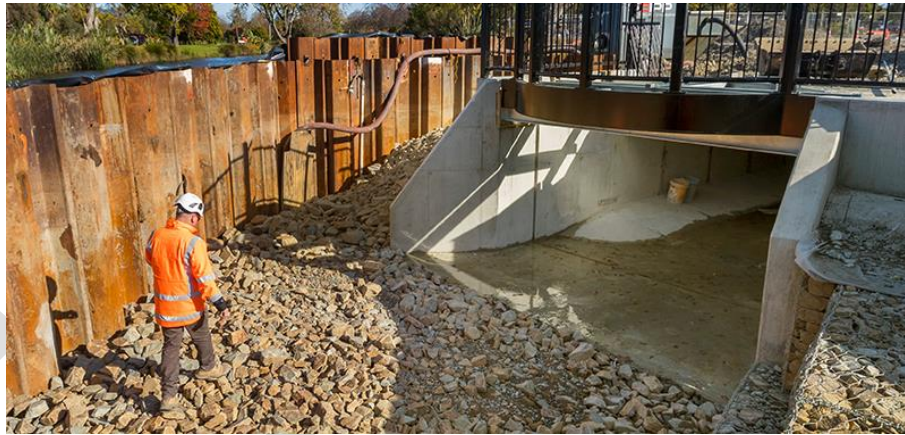
A control structure at a facility to provide storage to mitigate flood flows.
