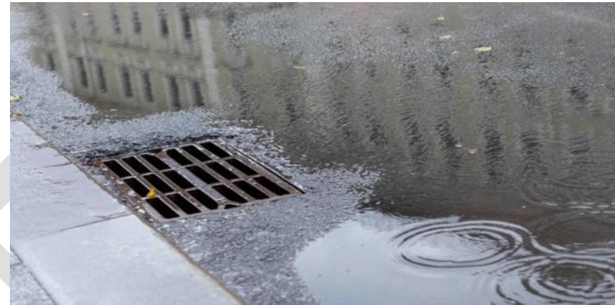
Example of land drainage
