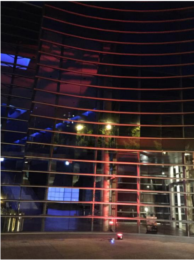
Figure 7-6: Trial of new in-ground forecourt lighting solution
