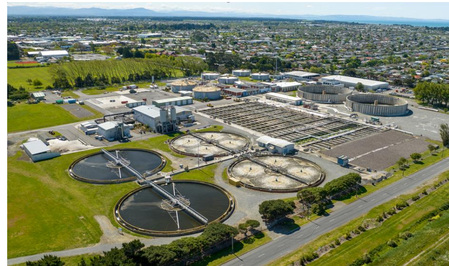
Christchurch Wastewater Treatment Plant.
