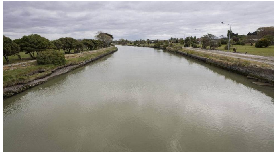
Stopbanks along a stretch of the Avon River will contain a tide associated with a one in 100-year storm. ( https://www.stuff.co.nz/the-press/news/125656079/avon-river-stopbanks-will-protect-area-from-one-in-100year-tide )
