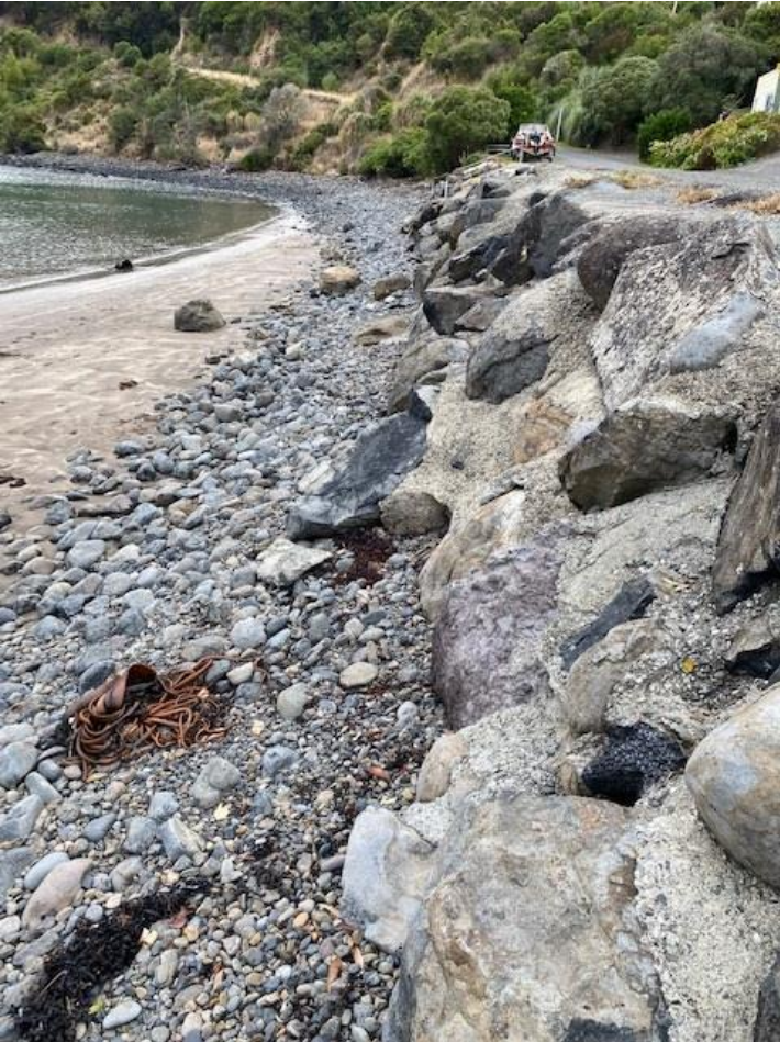
Photos 3, 4 and 5 - Seawall
