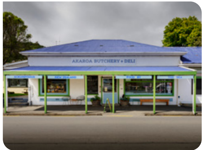
Figures 3 and 4 – Existing buildings on the site.
