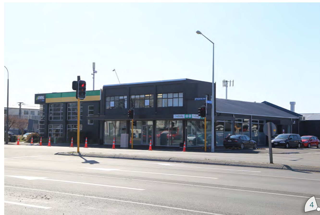
Photograph 4: View from the west of Fitzgerald Avenue looking eastwards
