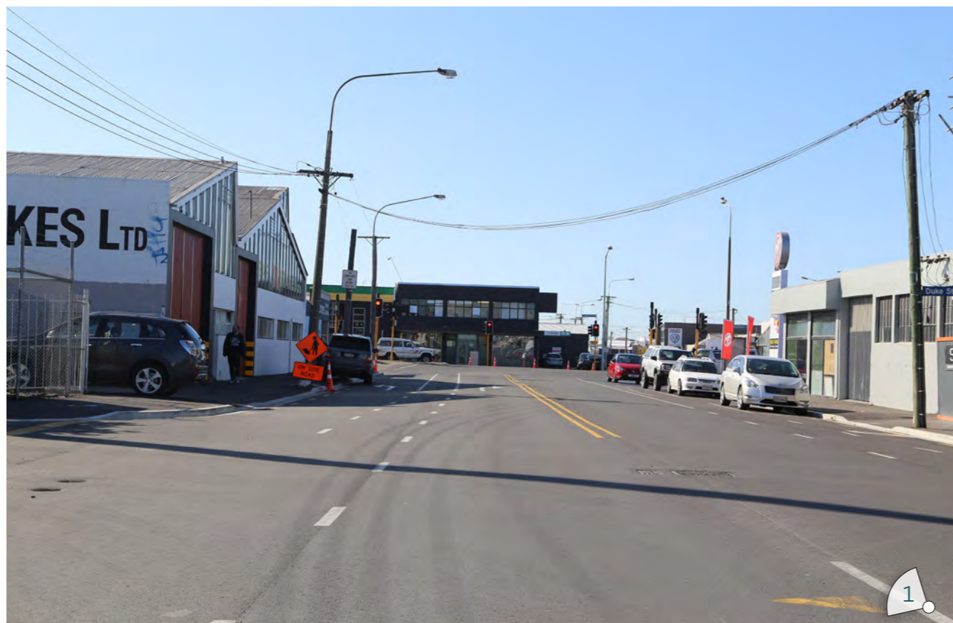
Photograph 1: View looking east along Tuam Street (approx. 60m to building)
