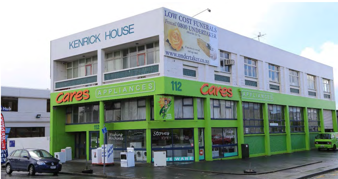
Image 4: The three-storey Kenrick House displaying a variety of signage styles is located just north of the Site
