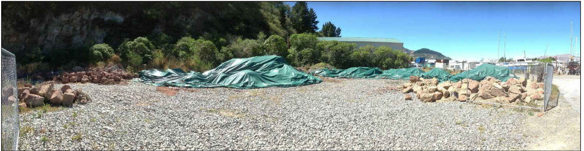
Photo 2: Tarp covered stockpiles
