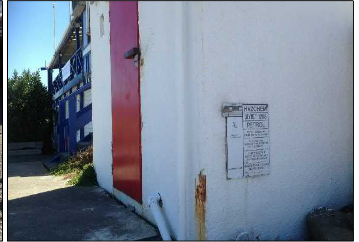
Photo 9: Underground fuel tank at the Coast Guard building
