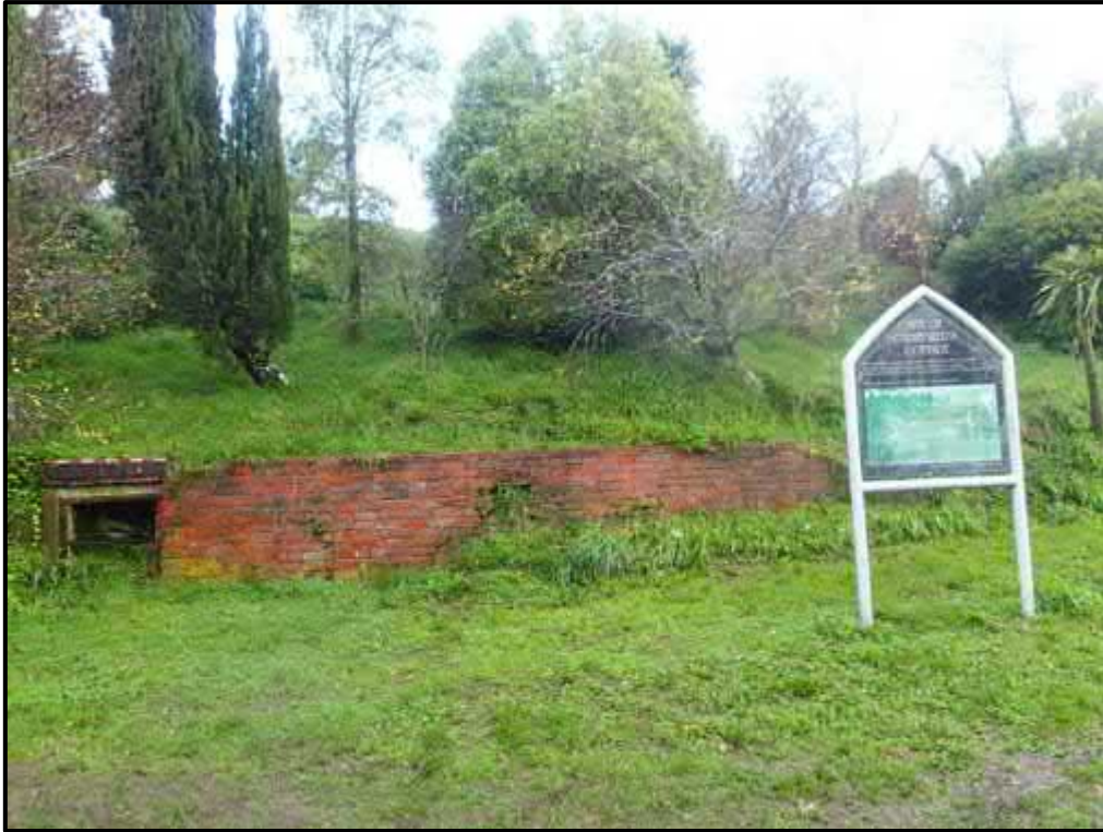
Figure 30. The Caretaker's cottage site, looking east, showing the brick retaining wall.
