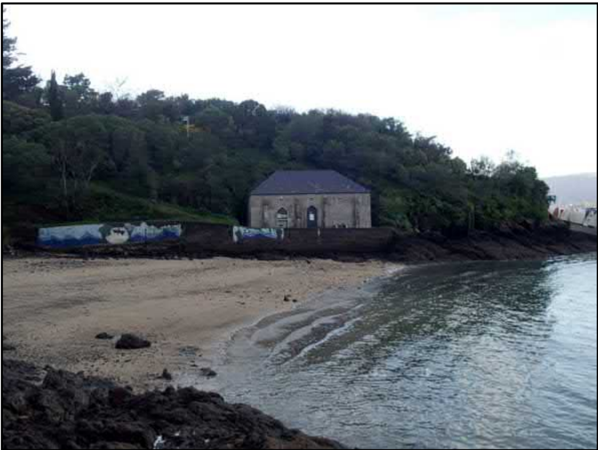
Figure 12. The 1874 magazine and seawall, June 2017.
