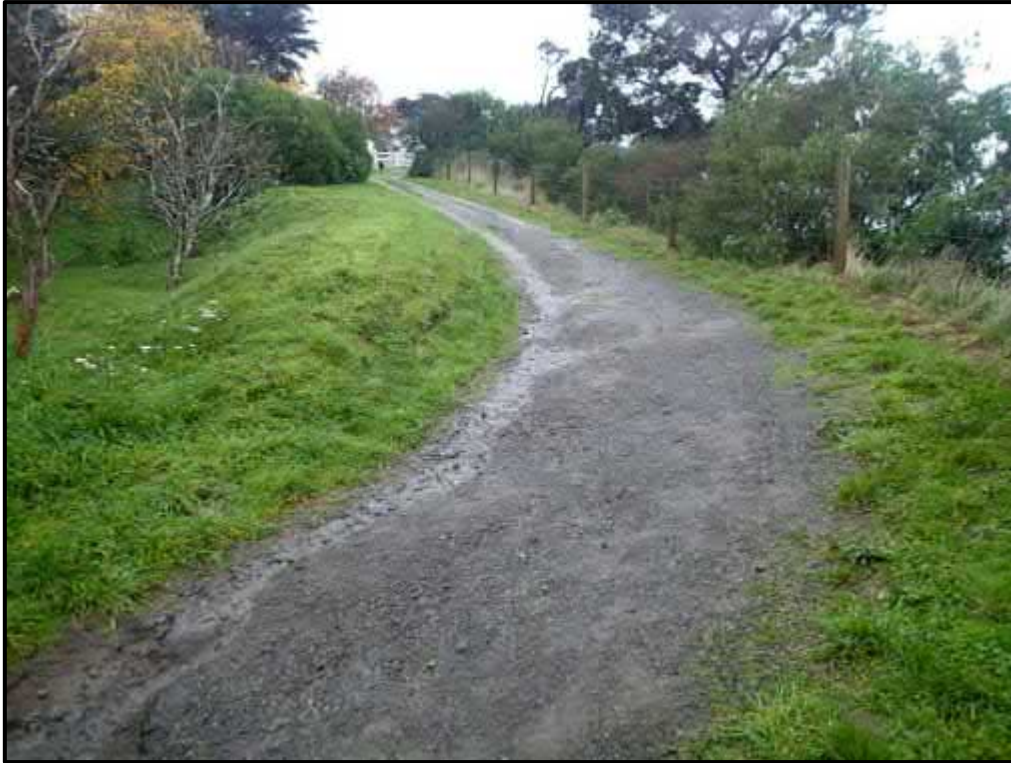
Figure 22. Looking north up the main vehicle/pedestrian access track, with the Park Terrace access gateway in centre distance. Raining at the time this photo was taken, note also the flow of water along the left hand side of the track, which has washed away the gravel in this location.
