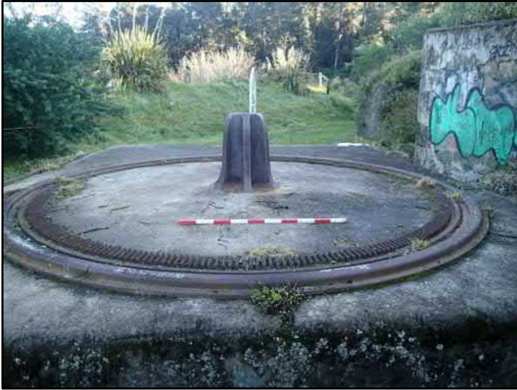
Figure 27. The Fort Erskine gun mount, looking north east.
