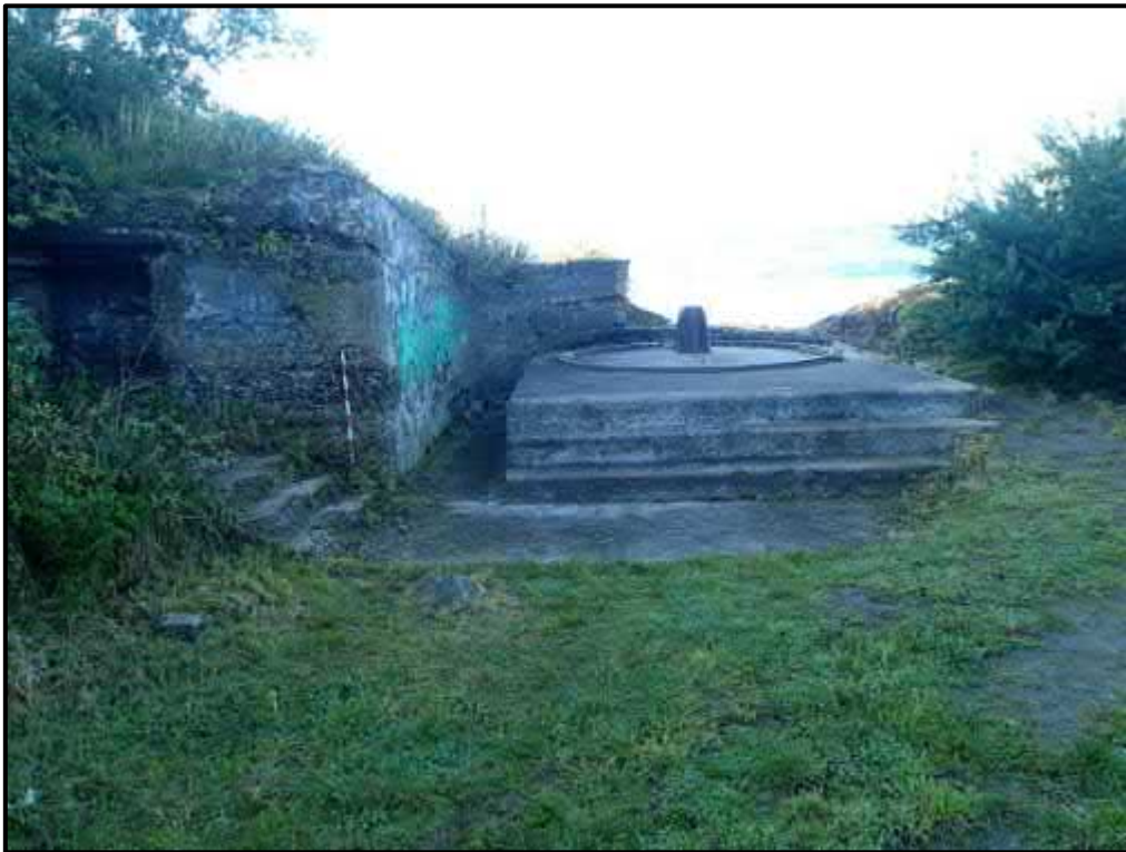
Figure 26. The Fort Erskine gun mount and surrounding concrete parapet wall, looking south east.
