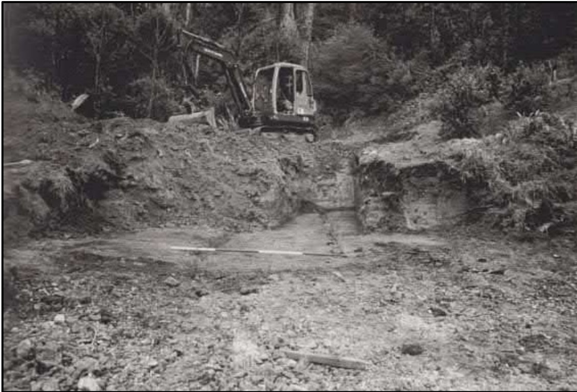
Figure 19. View of the 2002 torpedo boat shed excavation area, showing the asphalt/coal tar floor and timber rail bearers, looking north. Scale increments are 500 mm. Note the depth of fill. Image: Watson 2004: 11.
