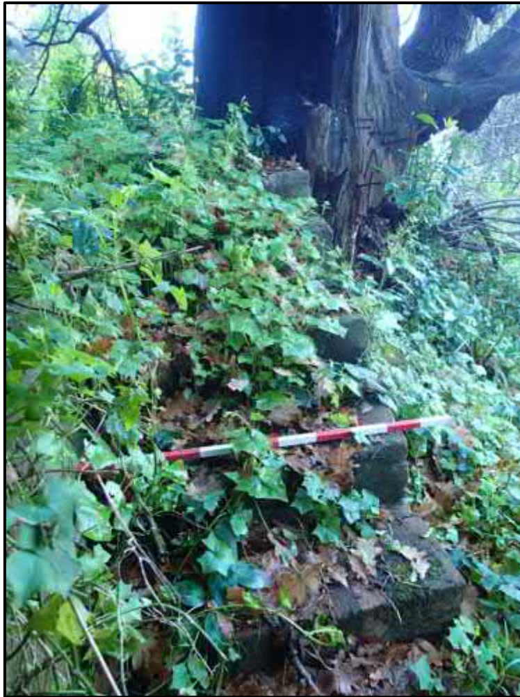
Figure 33. Brick steps located downslope of the caretaker's cottage site. These steps and an associated brick retaining wall are partially visible from the steps that lead down from the cottage site to the Magazine building.
