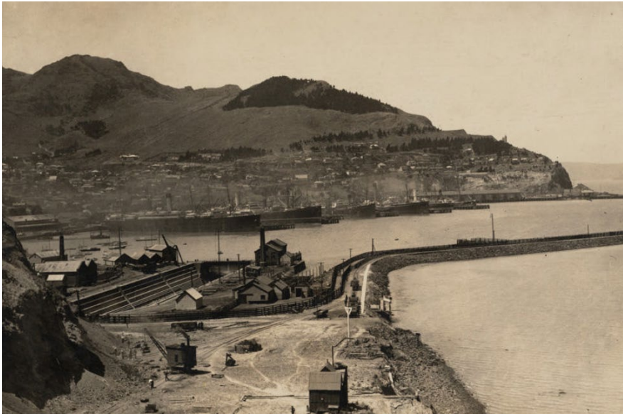
The cliff face being quarried for the wall around the reclamation, c.1911. (Image: Lyttelton Museum ref 14985.111).
