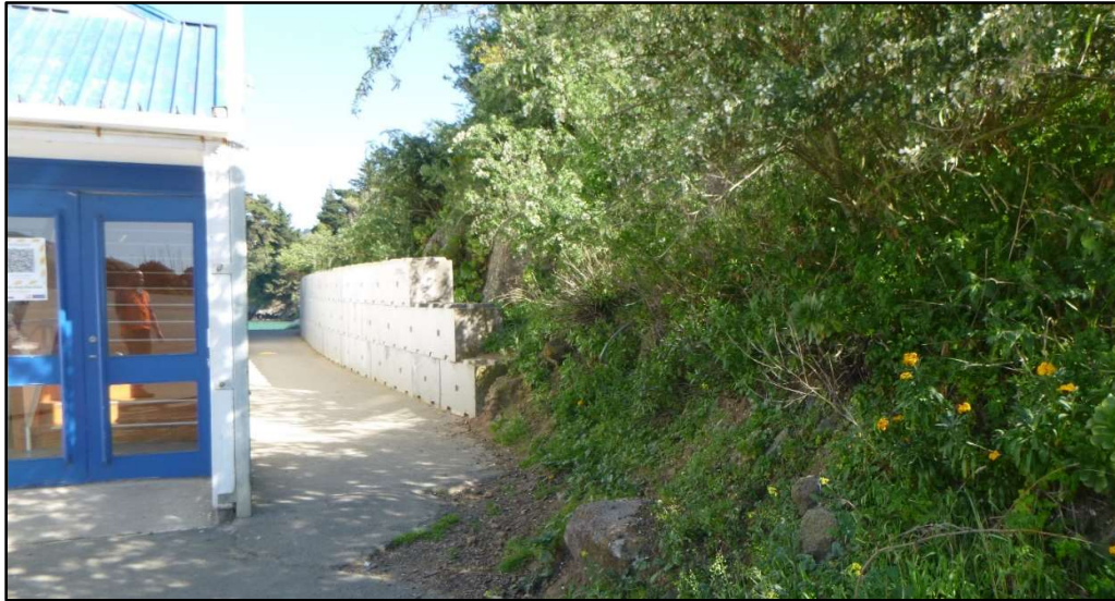
Figure 7 Concrete block wall behind the Yacht Club and the earth bund adjoining it on the right of the photo.
