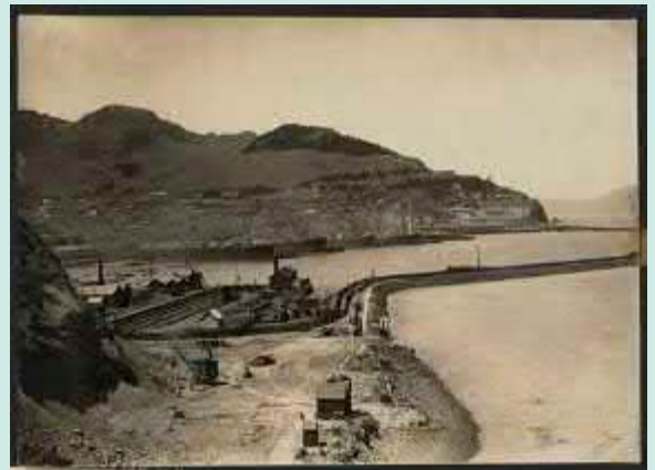
The cliff face being quarried for the wall around the reclamation, c.1911. (Image: Lyttelton Museum ref 14985.111).
