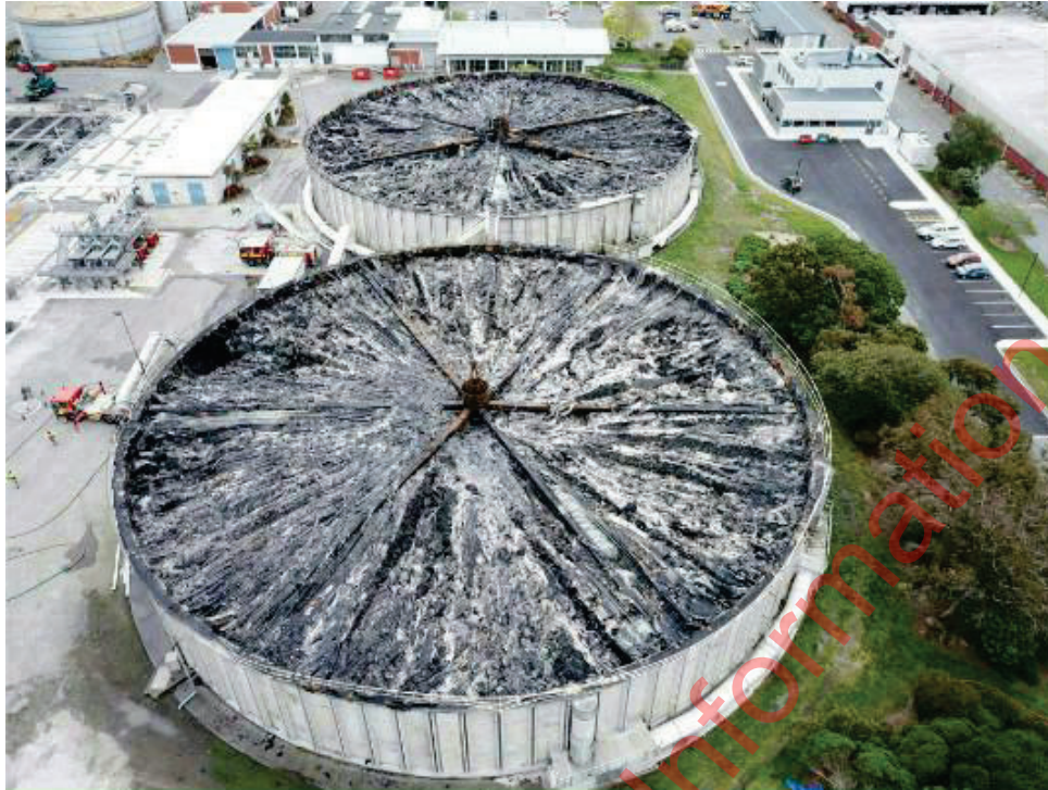
Photo 3: Aerial image of Tank #2 in the foreground. (Photo supplied by FIS from drone footage).
