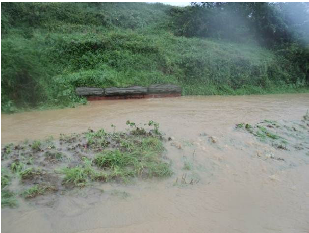
Figure 18 Truscotts Road at outlet of 1200 mm brick barrel
