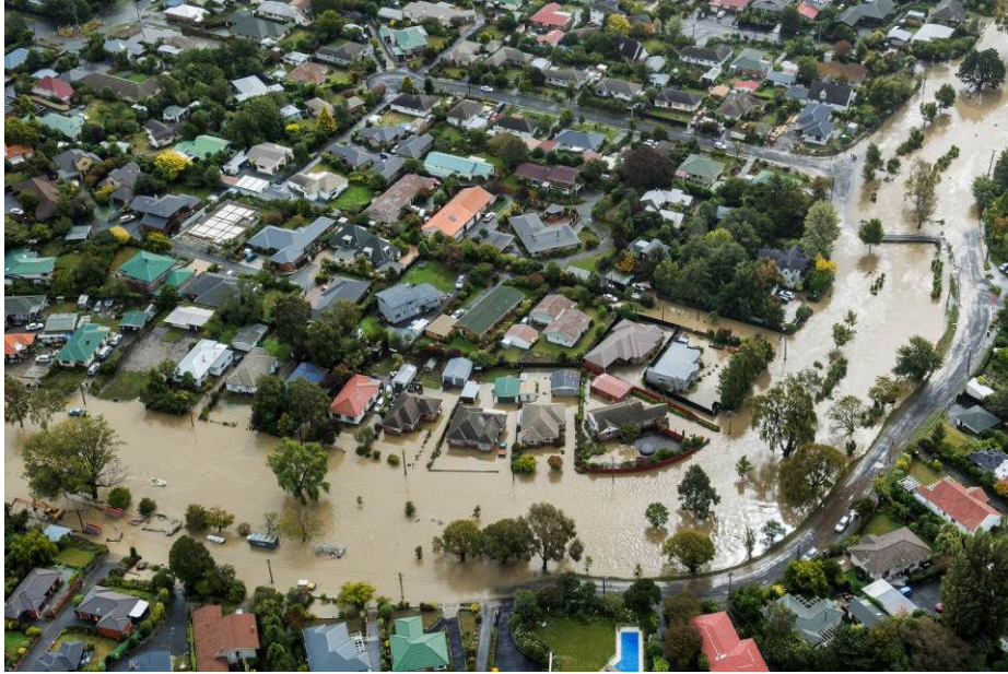
Figure 30 Extensive floor level flooding on Riverlaw Terrace
