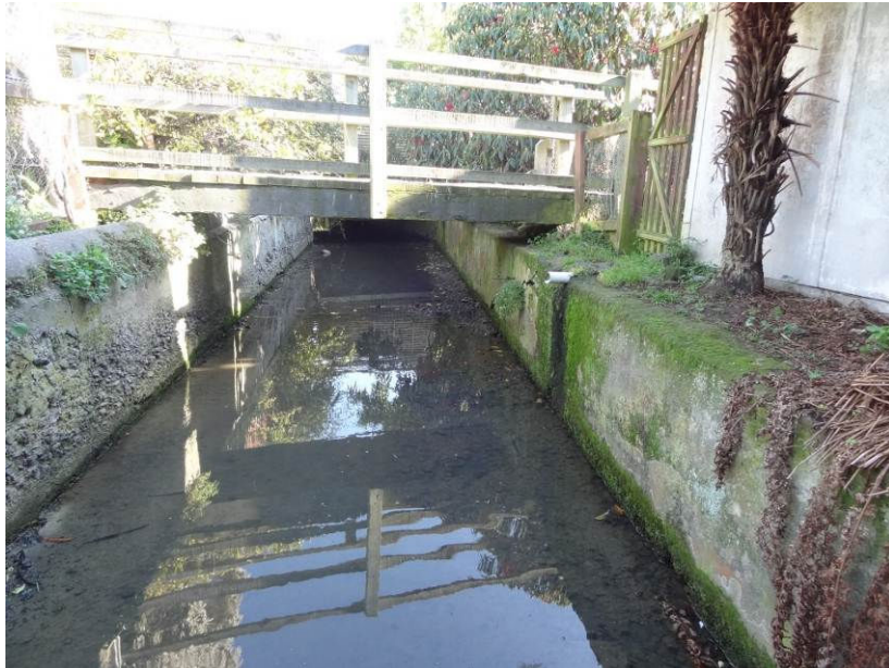
Figure 38 Sumner Main Drain with private access bridge
