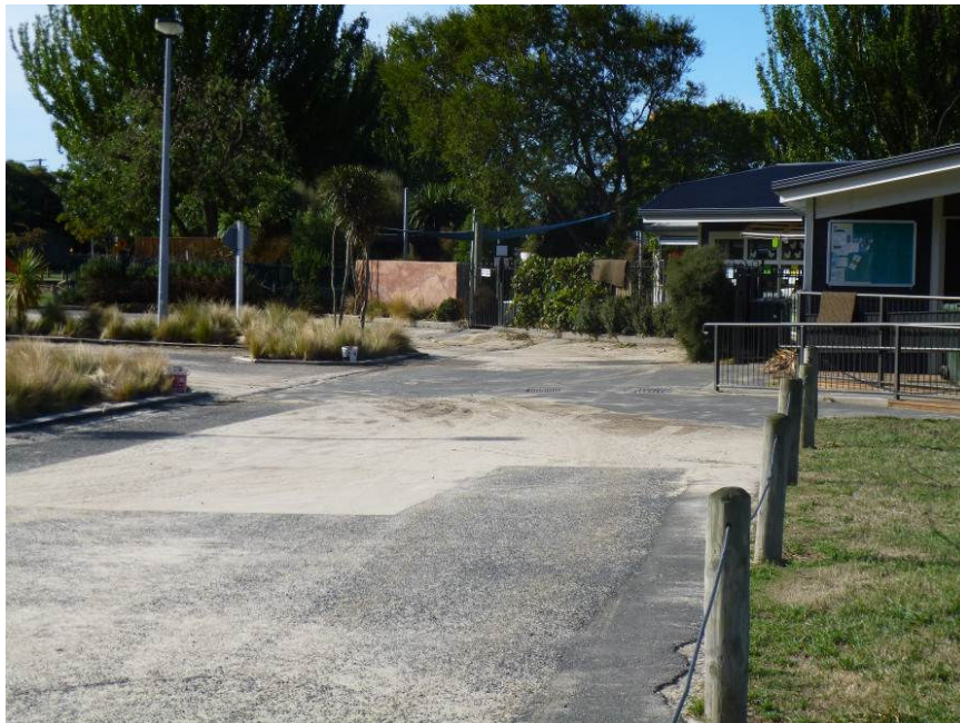
Figure 44 Moa Community Kids Early Learning Centre day after March 2014 flooding event
