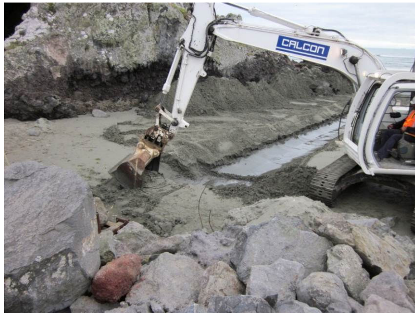
Figure 37 Cave Rock sand removal
