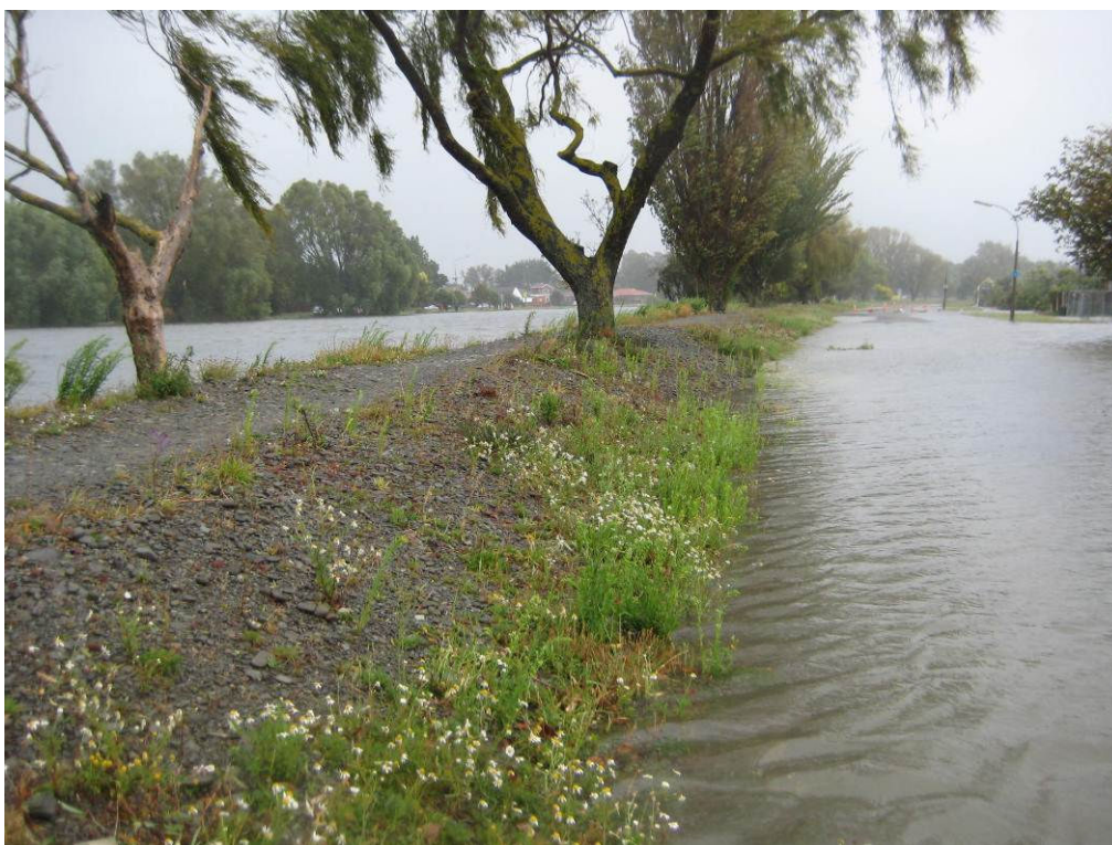
Figure 9 Lower Avon RRZ – flooding within stopbank
