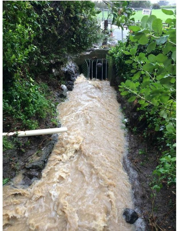
Figure 24 Bridle Path valley waterway - inlet at Port Hills Road
