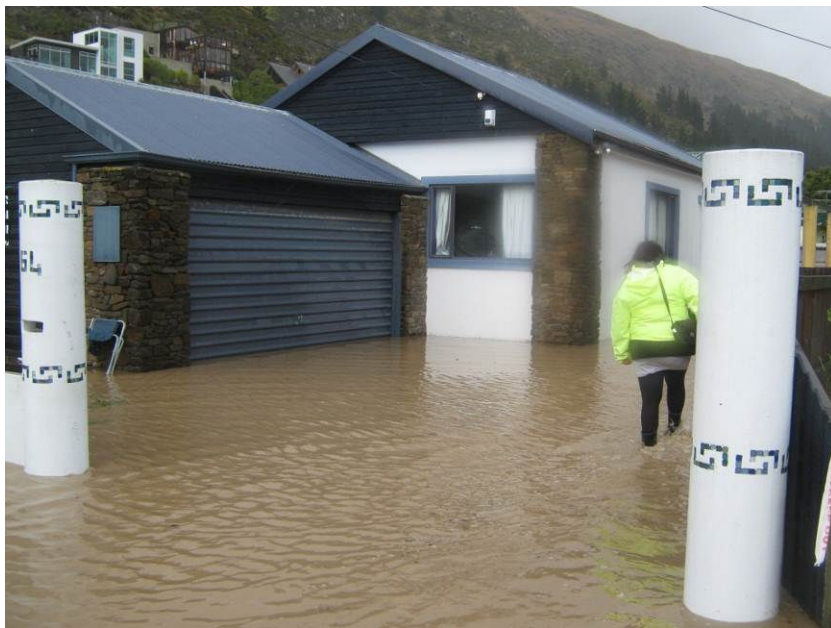
Figure 43 March flooding up to foundations
