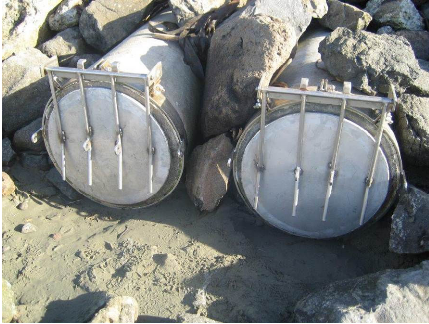
Figure 42 Burgess Street outfall with new flap gates
