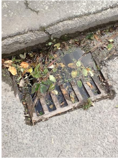
Figure 11 Brittans Drain sump two days after March 5th event
