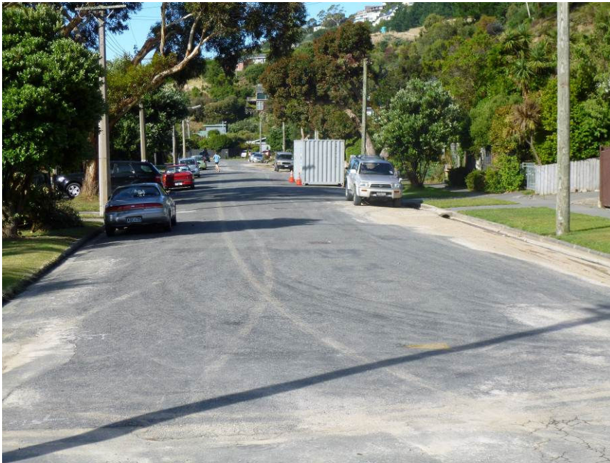
Figure 47: Top of Bayview Road with silt deposits day after March 2014 flooding event
