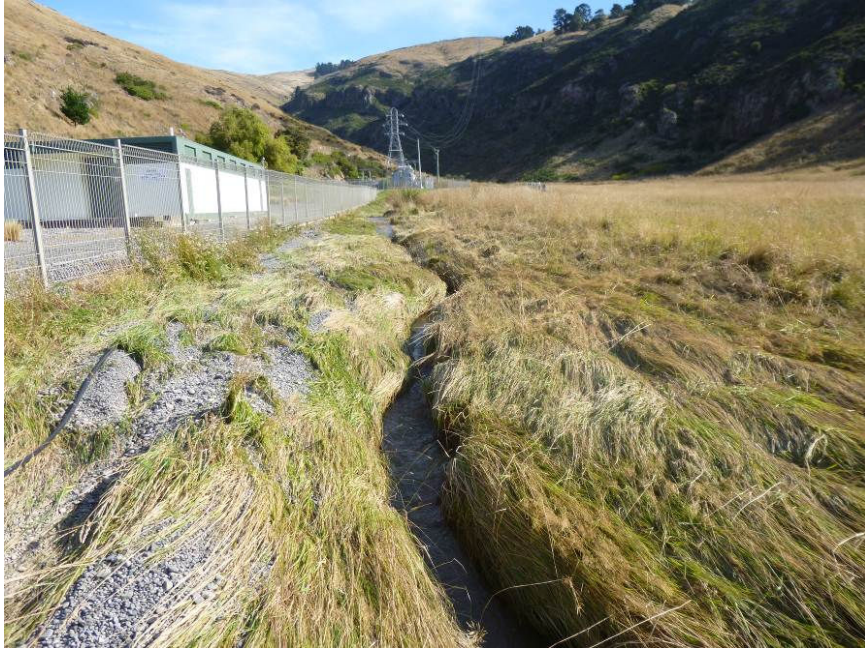
Figure 46 Rifle Range Drain in Barnett Park. High flood level indicated by flattened vegetation and gravel deposits
