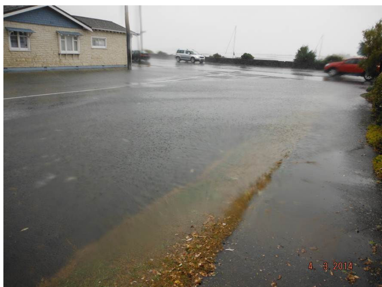
Figure 45 Surface flooding Bayview Road March 2014
