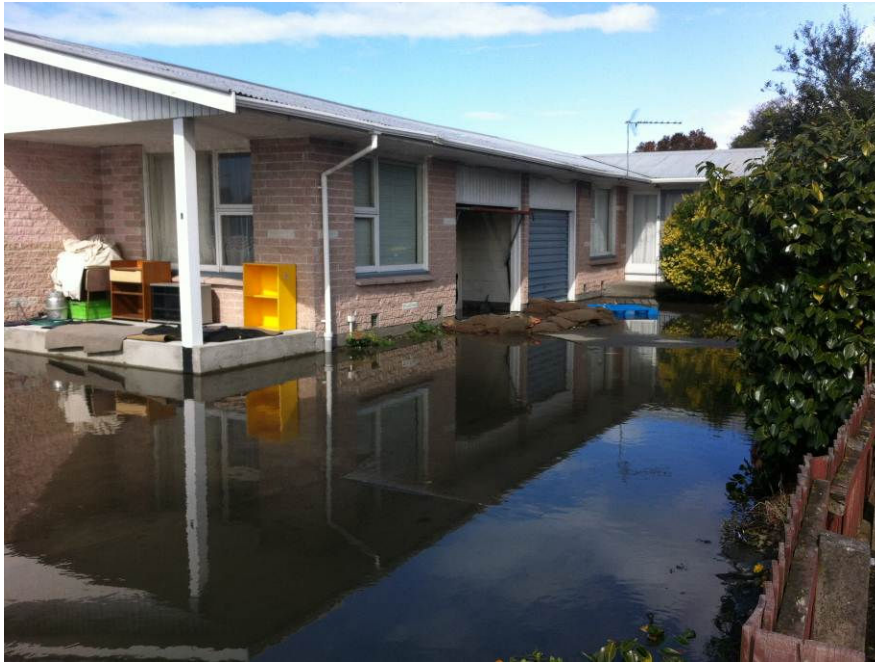
Figure 13 Ponding remaining around property three days after the March event
