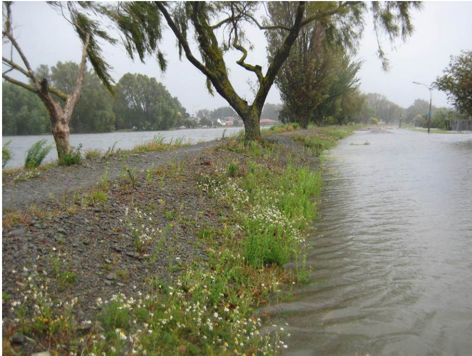
Figure 6 Lower Avon flooding behind stopbanks
