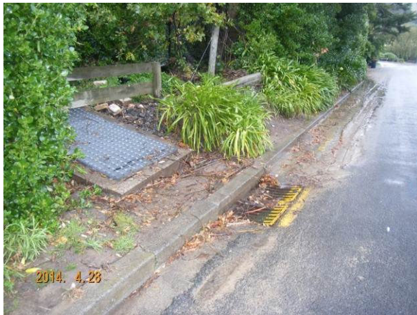
Figure 23 drain inlet structure at 78 Bridle Path Road
