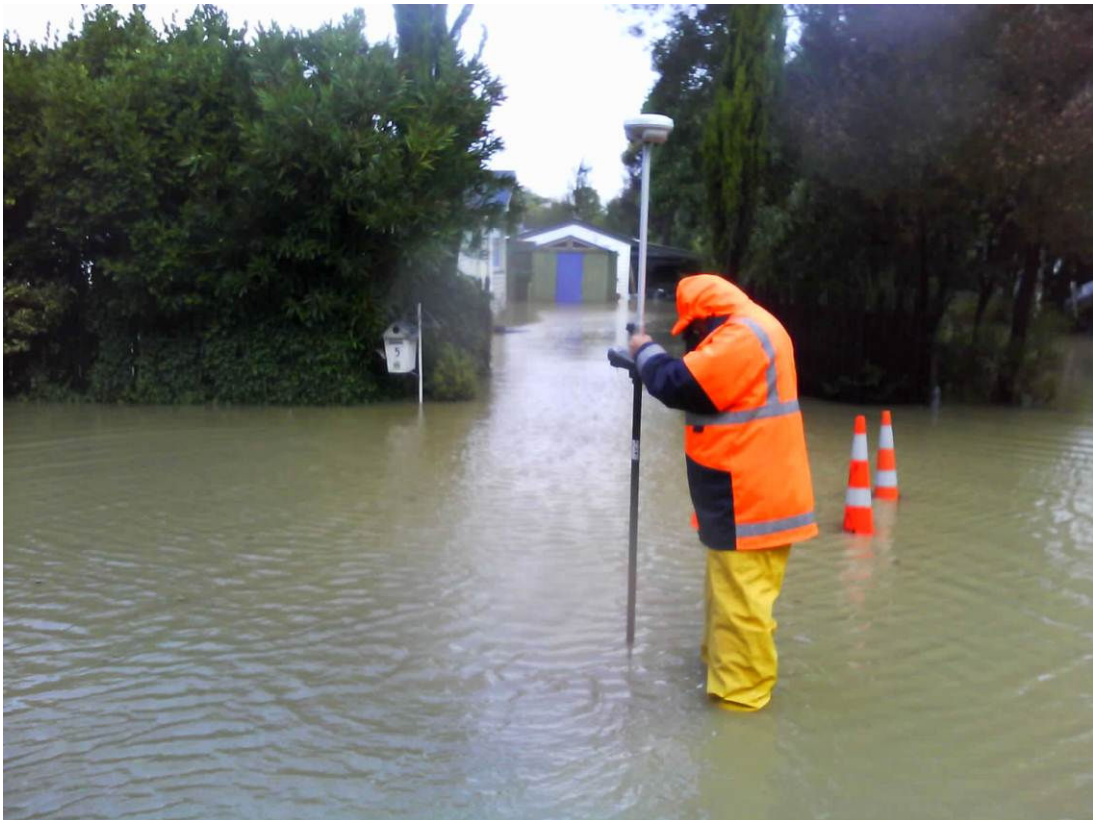
Figure 28 Lower Heathcote riverside properties - floor level flooding at Clarendon Terrace
