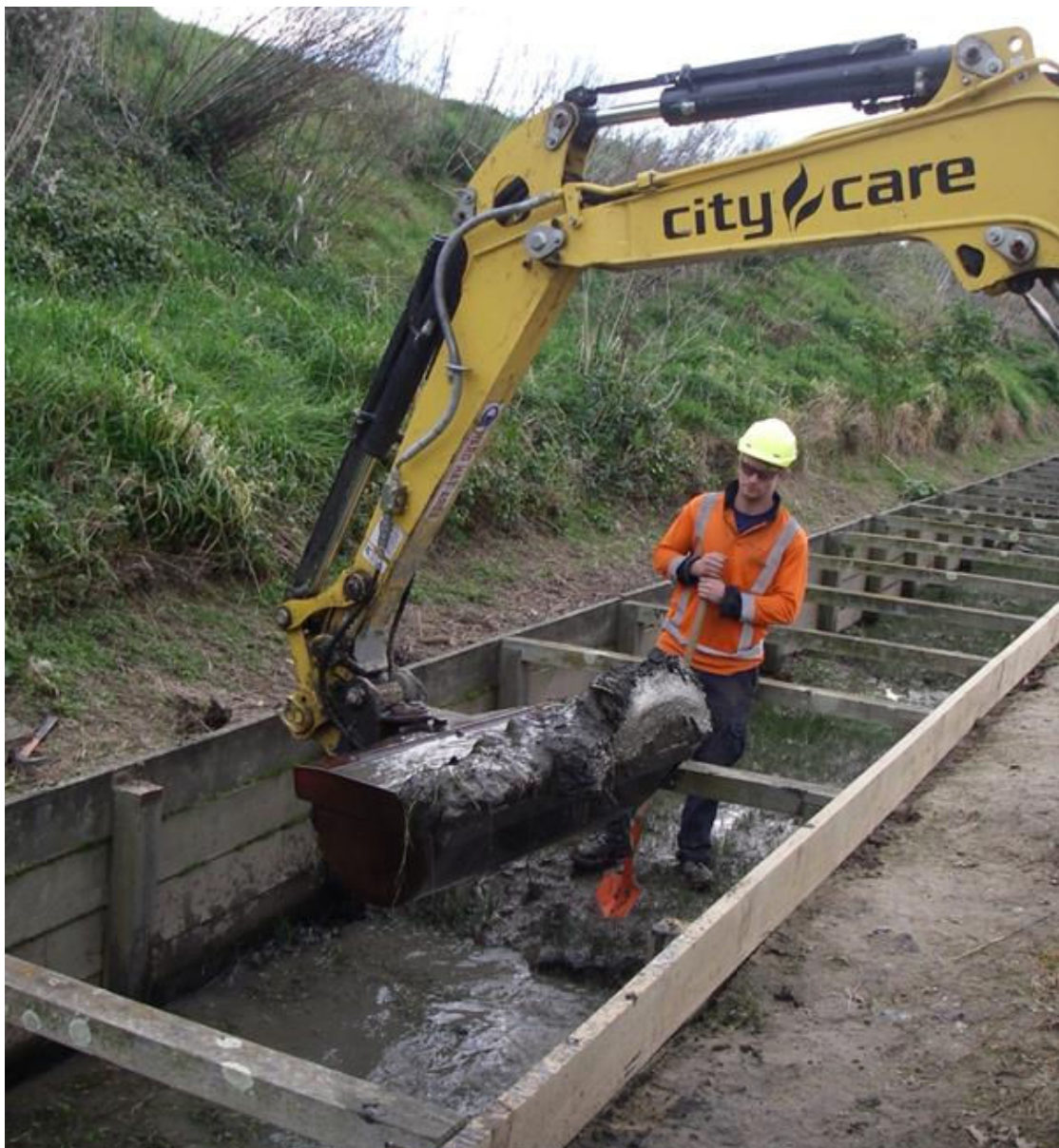
Figure 11 Maintenance in Truscott Drain July 2014
