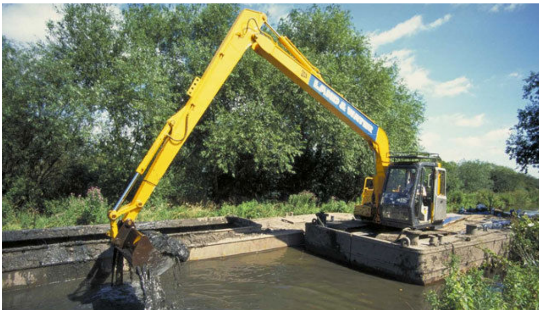
Figure 20 Dredging on a UK river
