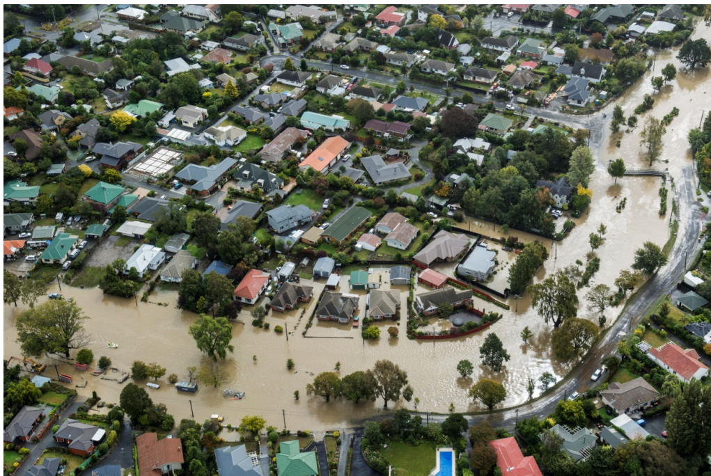
Figure 36 Lower Heathcote riverside properties - extensive floor level flooding on Riverlaw Terrace
