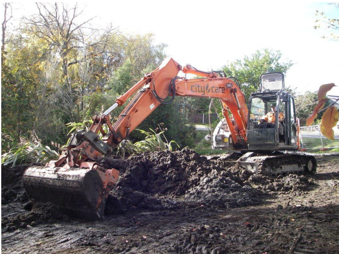
Figure 28 Maintenance works on Dudley Creek to increase channel capacity
