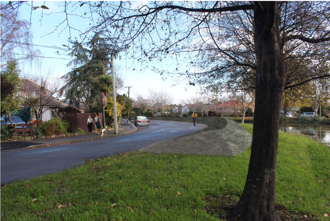
Figure 39 Concept image of aggregate stopbank along river
