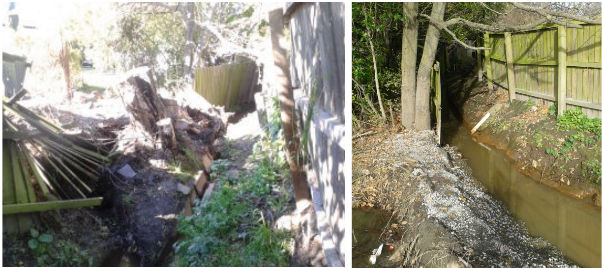
Figure 31 Brittans Drain before removal of tree (left) and after (right)
