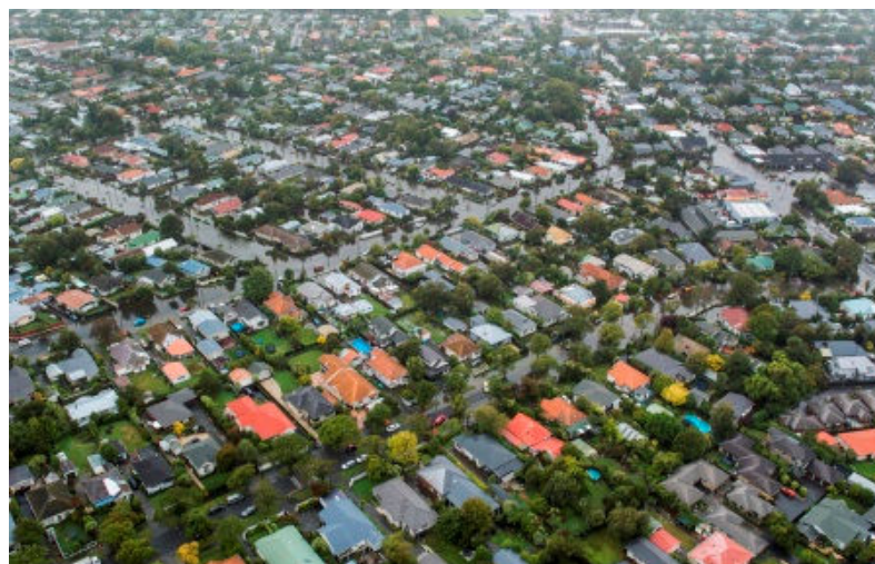
Figure 24 Flockton flooding in March 2014 event
