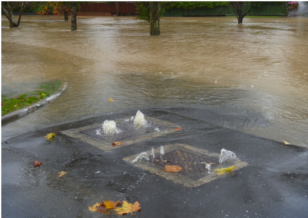
Figure 9 Wastewater overflow during a storm
