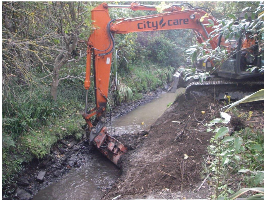
Figure 9 Maintenance works on Dudley Creek to increase channel capacity
