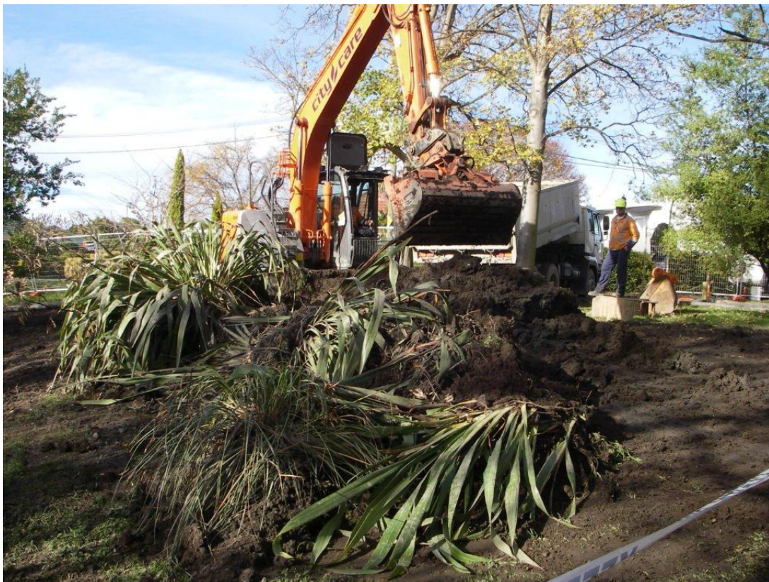
Figure 11 Clearing vegetation on Dudley Creek, May 2014
