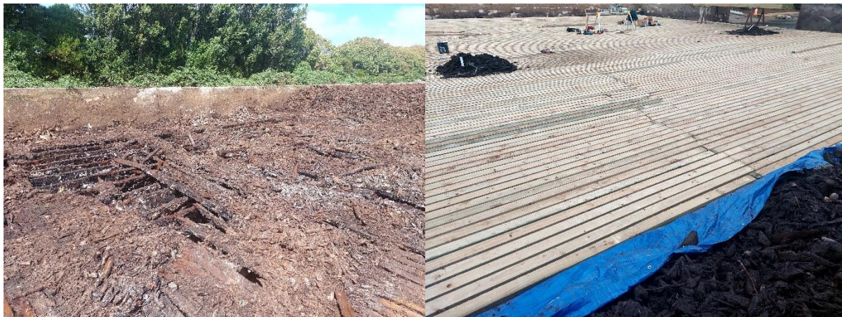
Figure 2.3: Wooden slat floor before (left) and after replacement (right) in 2023.
