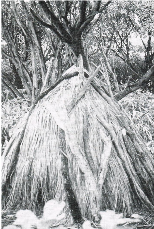
Example of a temporary shelter (whare rau) constructed of surrounding vegetation. "The branches are laid across the fern until they are melded together". 8
