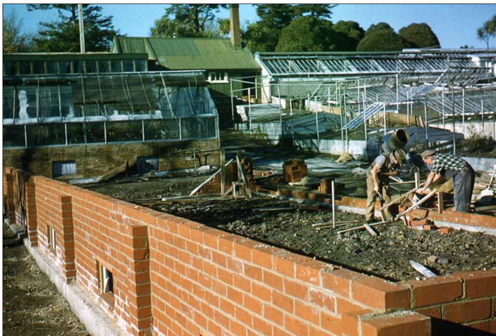
Figure 3.89. Construction works in the nursery area ca. 1957 Source: Flickr online image
