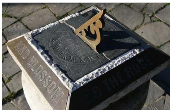
Figure 1.105. Slate dial plate and replacement gnomon. Source: L. Beaumont, 2010
