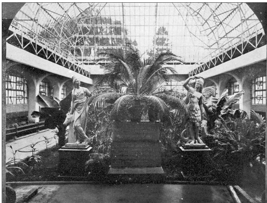
Figure 1.114. Cuninghame House interior with two of the Scott Statues c. 1924. Source: Historical photograph collection, Photograph 067, CBGP
