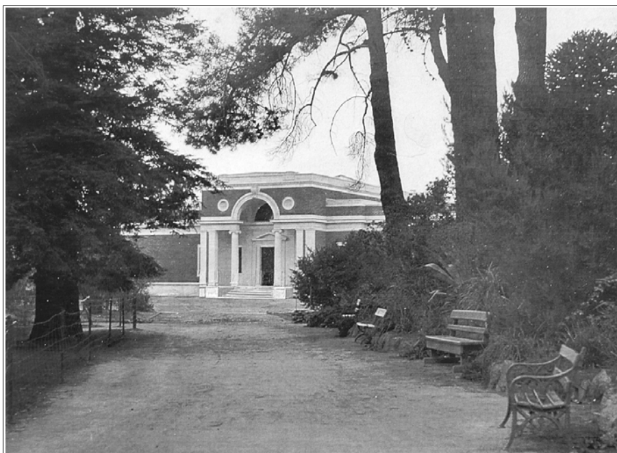
Figure 3.57. View of the newly completed gallery as seen from south walk bordering the Archery Lawn. Note the collection of seat styles placed alongside the walk.
