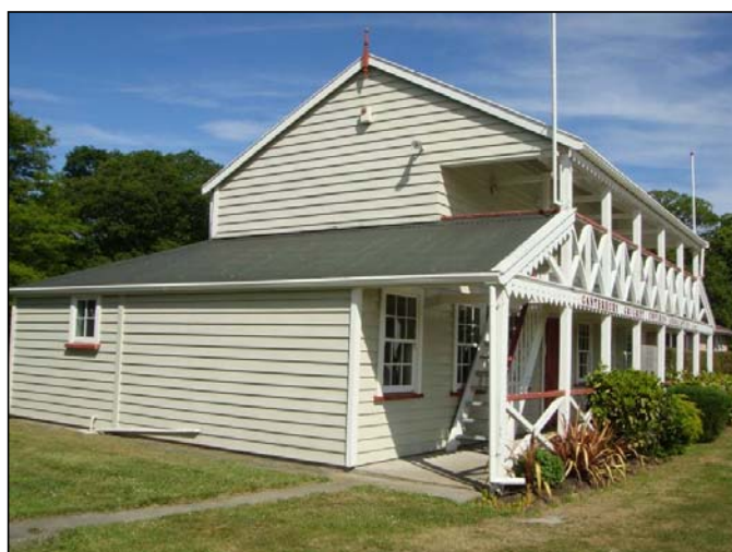
Figure 1.88. North-western view of the pavilion.
