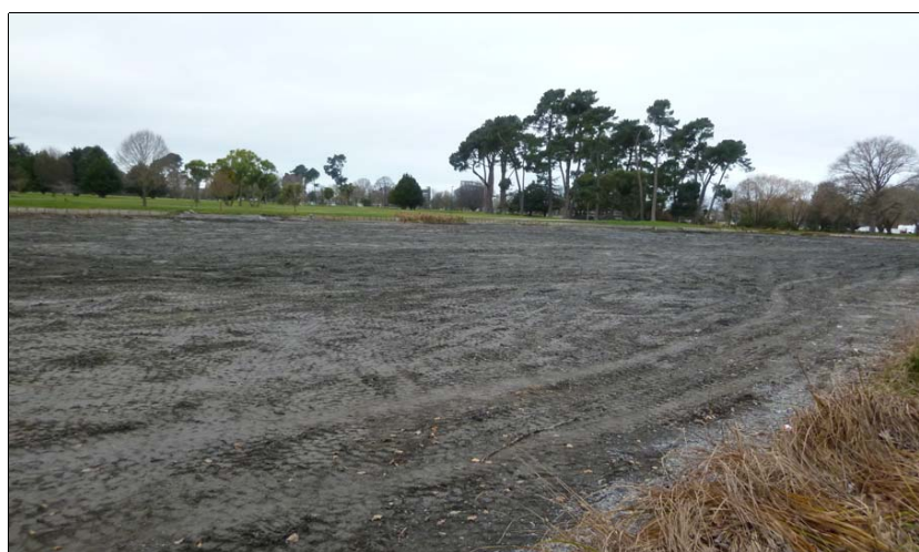
Figure 1.92. Lake Victoria drained post earthquake, August 2011. Source: L. Beaumont,
