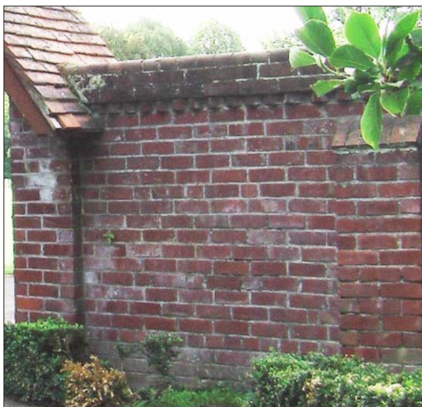
Figure 1.27. Boundary wall showing biological growth and initial stages of plant colonisation on brick surface. Source: L. Beaumont, 2012
