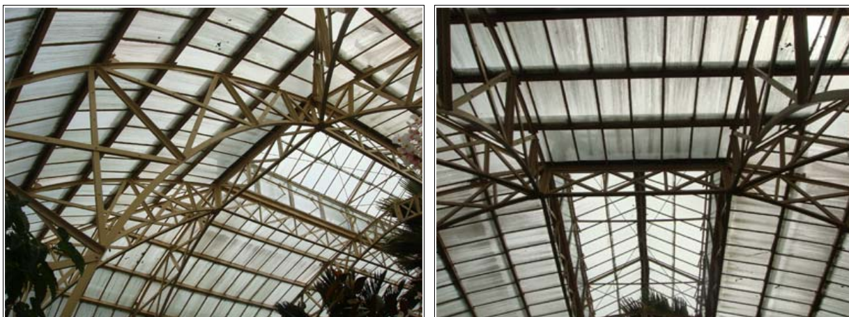
Figure 1.63. The roof structure with large steel trusses and the steel purlins.
