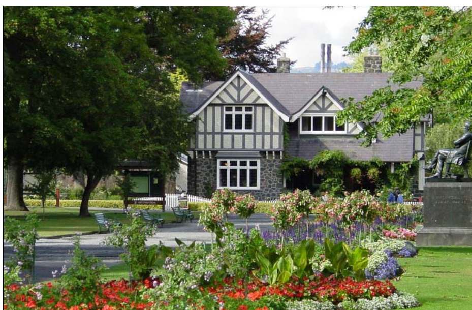
Figure 1.44. Curator's House following repair and strengthening. Source: Christchurch City Council, Future Christchurch
