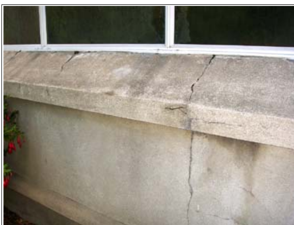
Figure 1.69. Cracks in the plaster spandrel (left) and in the windows sills extending down the wall (right).
