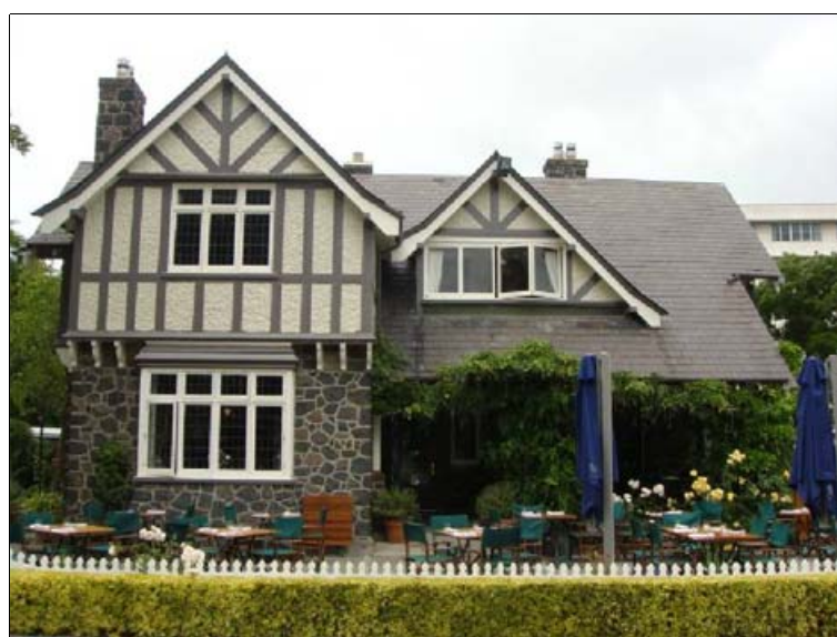
Figure 1.47. L-shaped northern elevation with gabled dormer above the verandah. Source: DPAL
