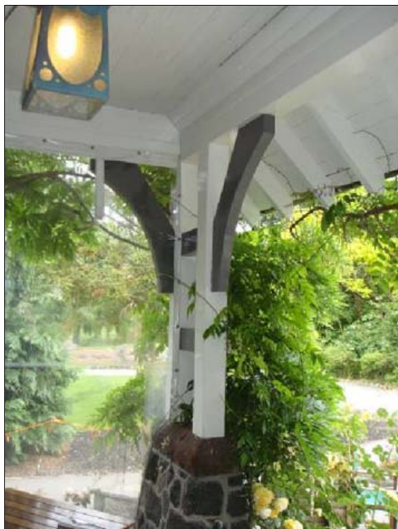
Figure 1.46. Verandah posts. Source: DPAL
