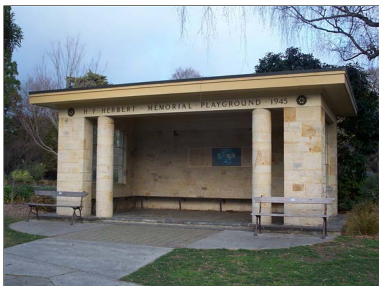
Figure 1.42. Pre-earthquake view of Pavilion. Source: L. Beaumont, 2011
