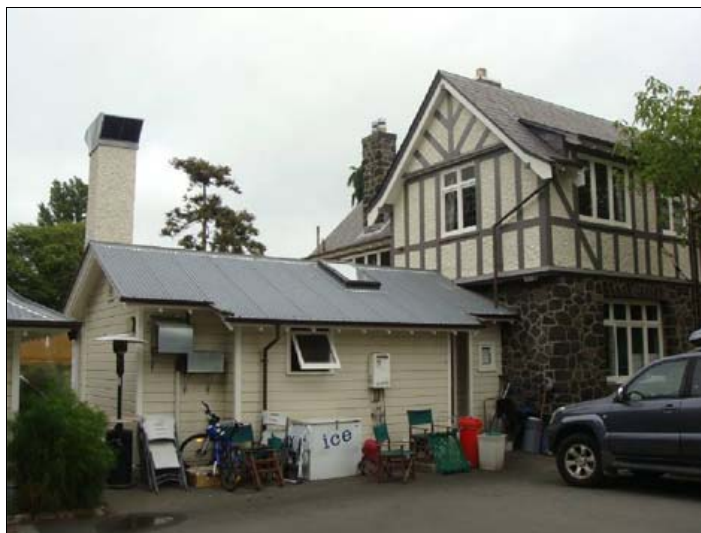
Figure 1.49. Extension on southern side of eastern elevation. Source: DPAL
