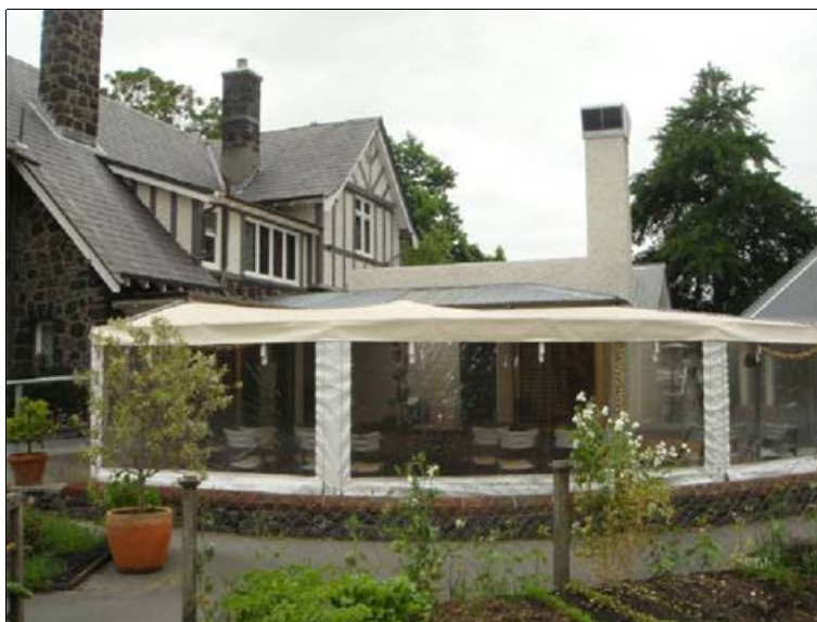
Figure 1.50. Looking towards the southern side of the house from the west. Source: DPAL
