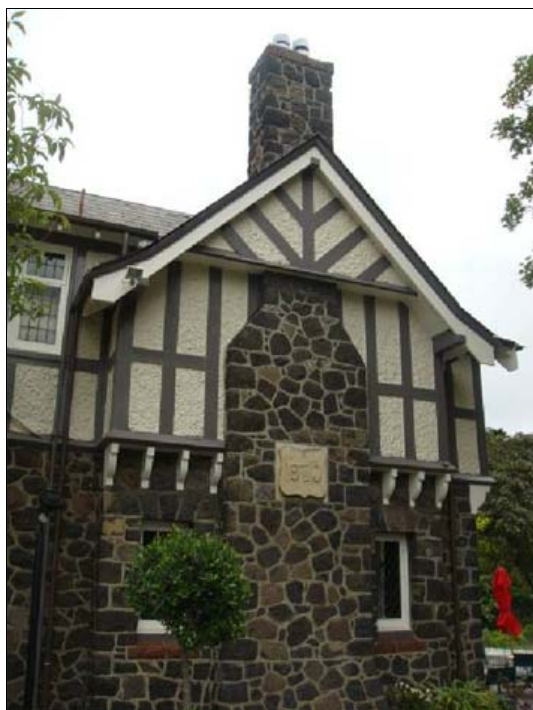
Figure 1.48. Chimney breast on eastern elevation. Source: DPAL
