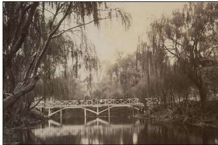
Above: College Bridge and Hagley Park, March 1880 Source: O.027000, MNZ
