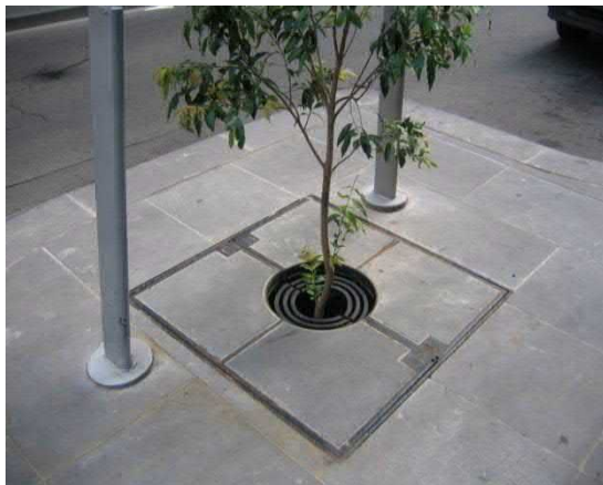
Little Burke Street, Melbourne
