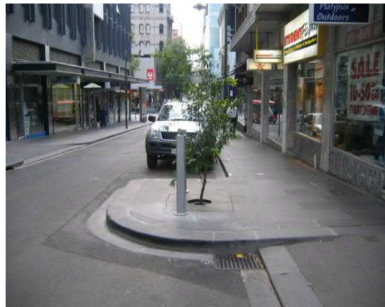
Little Burke Street, Melbourne
