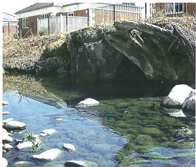
Figure 9-12: Large stumps placed upside down on the outside of a bend will create a stable overhang, and create an interesting landscape feature. An area of deeper water under the stump will provide excellent cover for fish. Papanui Stream above Grants Road, 2002.
