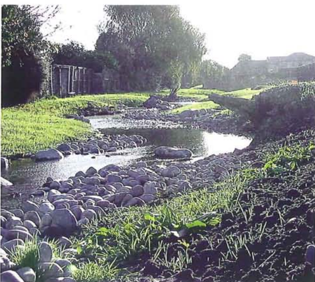
Figure 9-7: If creating a vertical bank, ensure that the opposite bank is shallow to prevent channel incising and to allow accommodation of flood flows. Newly restored Papanui Stream above Grants Road, still to be planted.
