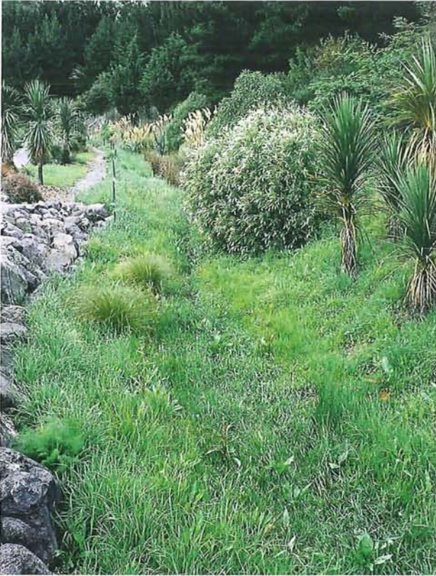
Figure 7-6: Planting grass in the waterway channel and vegetation on the bank is a soft alternative for bank and channel stabilisation. Glenstrae Stream at Drayton Reserve.
