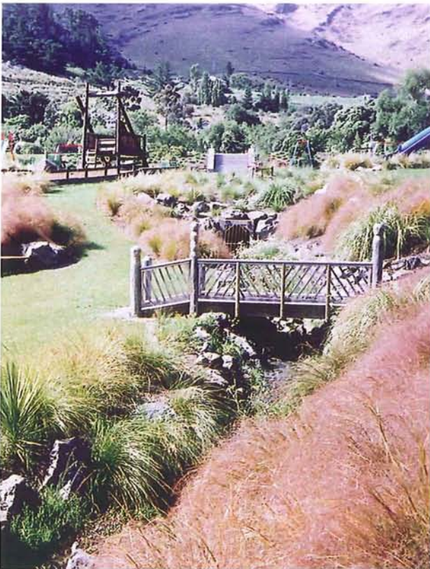
Figure 7-9: The combination of structural methods of bed and bank stabilisation (rockwork) with softer vegetative methods have created a natural looking hill waterway, structurally able to withstand flood flows. Bridle Path Stream at Heathcote Domain.
