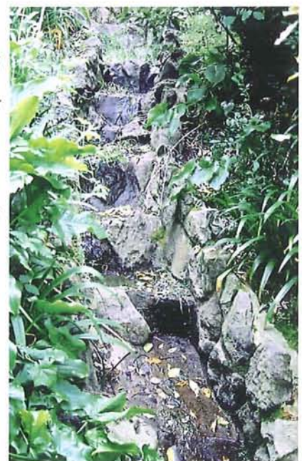
Figure 7-5: A series of properly designed cascading drops and pools will dissipate water flow energy and so reduce the erosive power of the flow. The growth of vegetation along the waterway banks will help to soften an otherwise hard structure. Unnamed Stream, Augusta Street.
