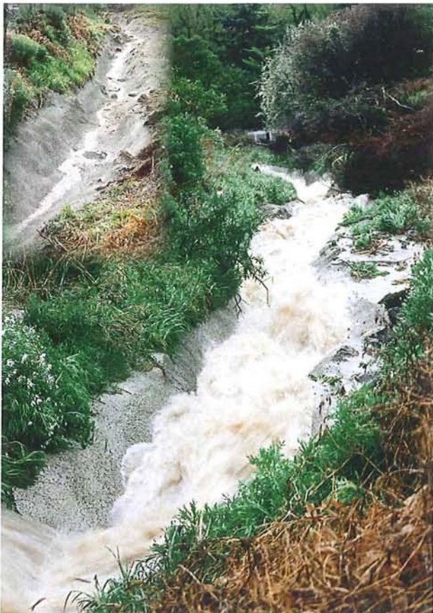
Figure 7-7: Smooth, steep, concrete cast channels result in fast, unmanageable water flows that are not acceptable for hill waterways.
